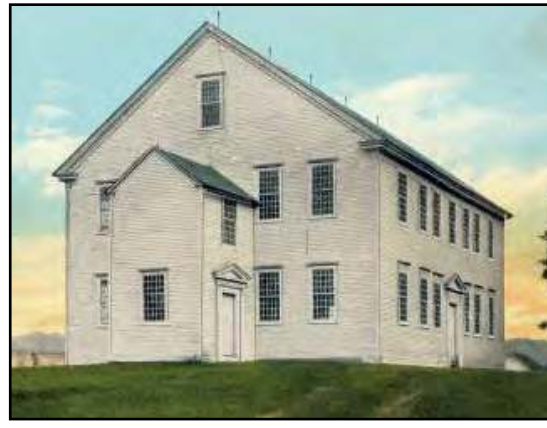
Rockingham Meeting House, built in 1787. PHOTO PROVIDED
