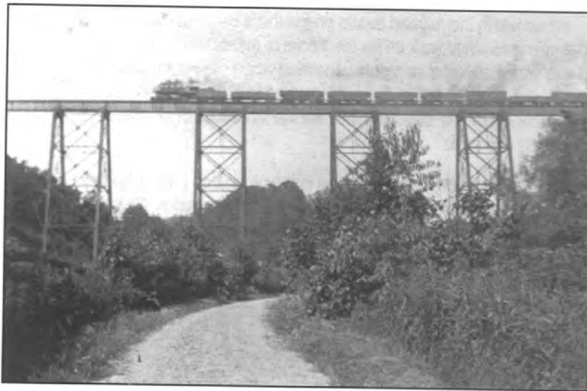
STARTING in 1911 NYC freight trains crossed Tinkers Creek Valley on this trestle-supported bridge. (Date of photograph unknown. Photo reproduced by Nina Wolf)
