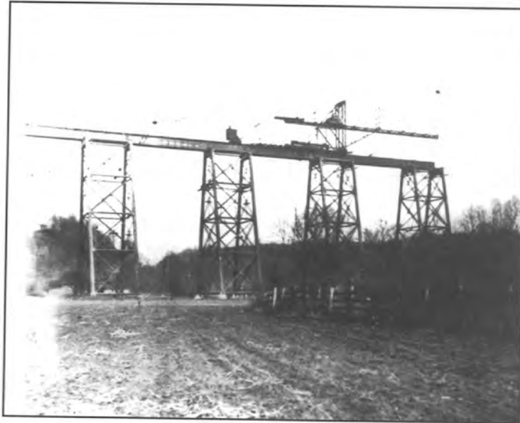
CONSTRUCTING THE NYC TRESTLE BRIDGE over the Tinkers Creek Valley. (Photo reproduced by Nina Wolf)
