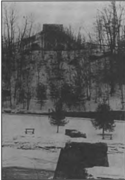
The SOUTH TRESTLE ABUTMENT as seen from Hemlock Creek Picnic Area. (1994 photo by Judi Schroeder)
