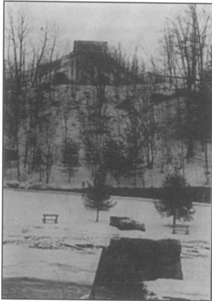
The SOUTH TRESTLE ABUTMENT as seen from Hemlock Creek Picnic Area. (1994 photo by Judi Schroeder)
