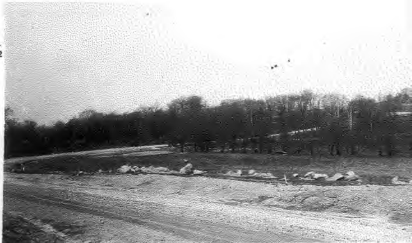
Before they built their new home in Walton Hills, Jack and Mary Bell took this photo of their building site at 17455 South Meadowpark Drive. (early 1950s photo)
