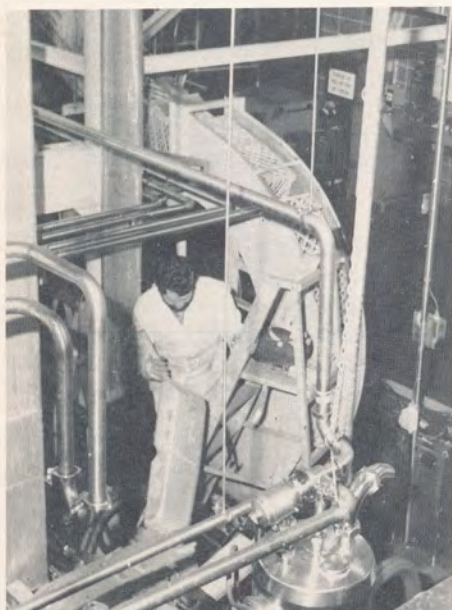
Henry Ricard installs piping during production downtime.
