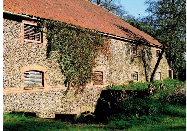
Letheringsett, Norfolk: part of the west front of the mid-18th-century 40-coomb malthouse in the brewery yard; with the kilns it is 45 metres long [photo Margaret Bird 2001]
