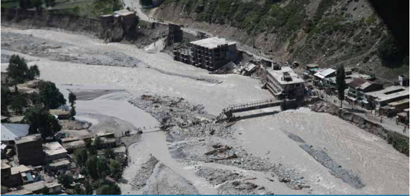
Damaged bridge from flooding, Pakistan. Photo © Wikimedia/Horace Murray
