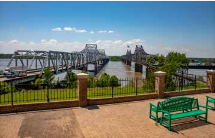
Top: New LED roadway lighting was installed. Bottom: The bridge was opened in 1973 and is next to the Old Vicksburg Bridge, which opened in 1930 and is now exclusively a railroad bridge.
