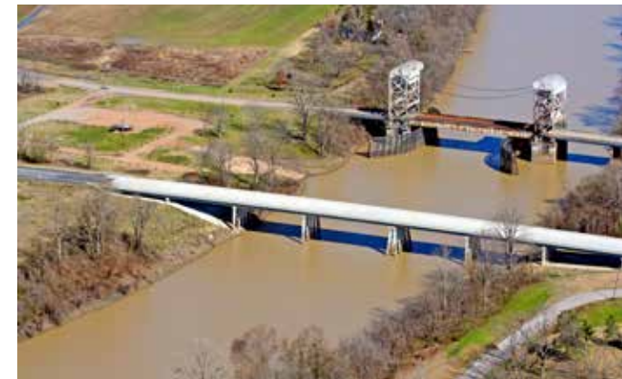
Top: TIMED provided critical facility improvements to the Port of New Orleans.
