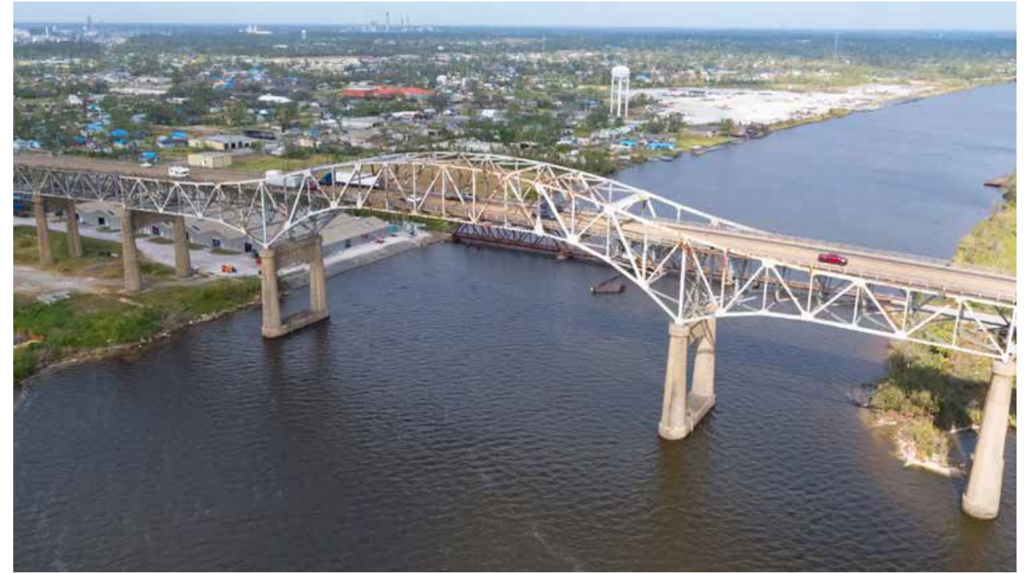
The Calcasieu River Bridge has been a southwest Louisiana landmark since 1952.
