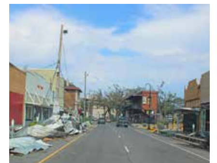
Extensive damage along LA 24 in downtown Houma after Ida.
