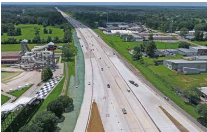
Construction on I-10 at Highland Road in 2020.
