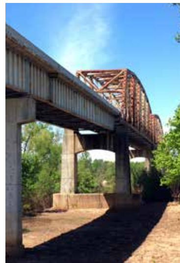
The Jimmie Davis Bridge over the Red River in Shreveport.
