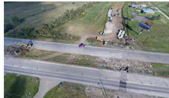
Above: The future intersection of the new roadway and LA 3235.
