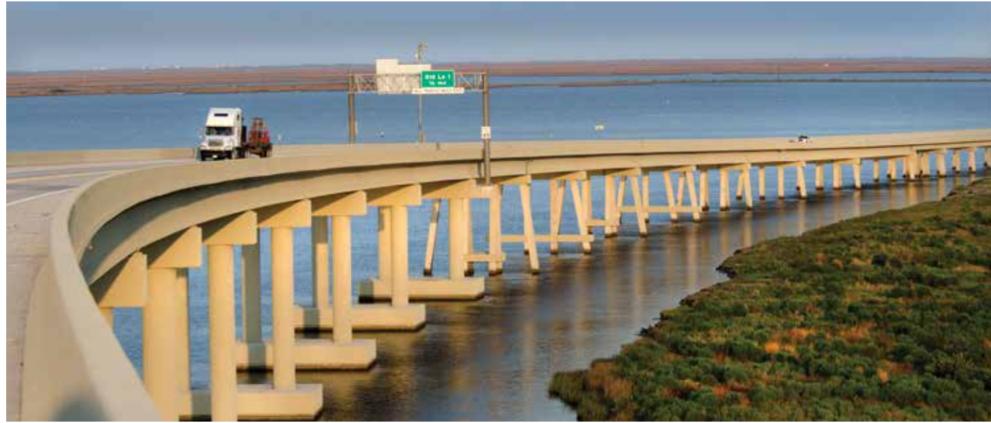
LA 1 high-rise bridge over Bayou Lafourche in Leeville.
