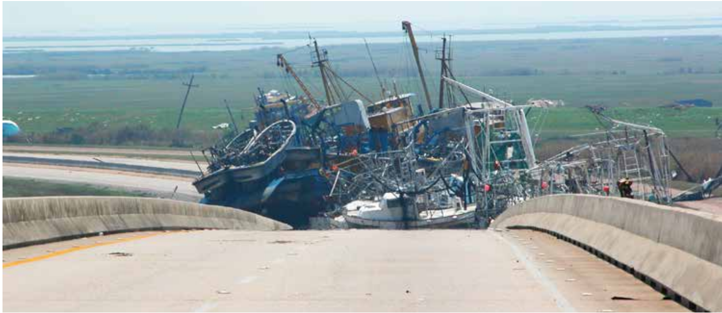
A jumble of boats on LA 23 in Empire following Hurricane Katrina in 2005.
