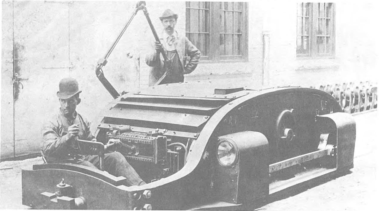
Two-ton electric mining locomotive.
