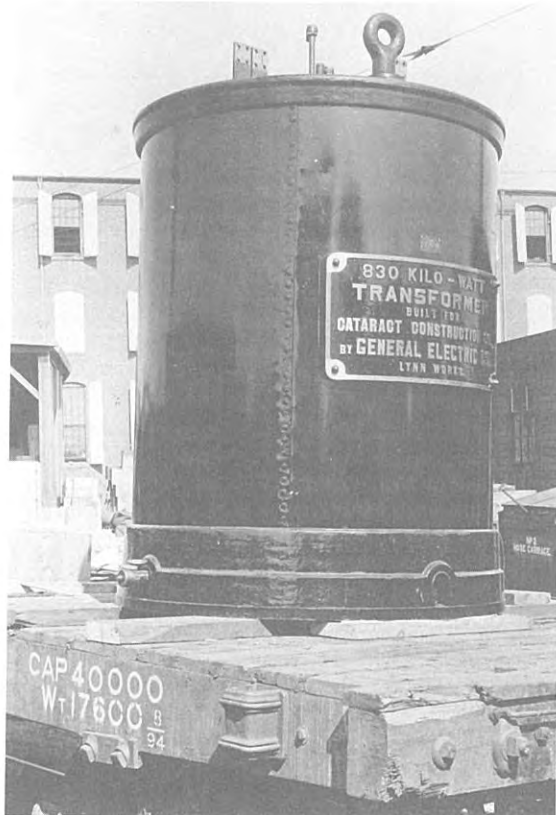
Transformer for the Niagara Falls hydroelectric station — 800 kw, 10,000 volts.
