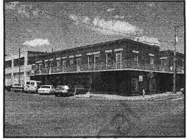
Figure 5:20. 315-317 W. Overland. Franklin Grocery and apartments. NRS building in background.
