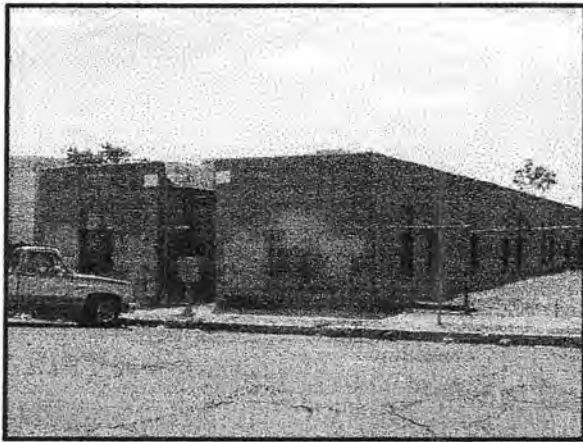
Figure 5:25. Motor Supply Building built 1930. 308 Chihuahua
