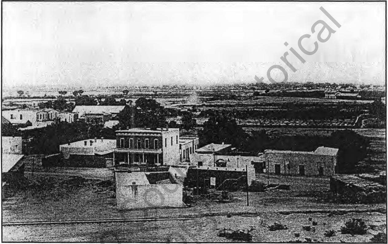
Figure 2:9. This picture shows the present site of the Aronstein-Stevens Building corner of San Francisco and South Santa Fe Streets. The white adobe house with the high wall is the old J.P. Hague home.
