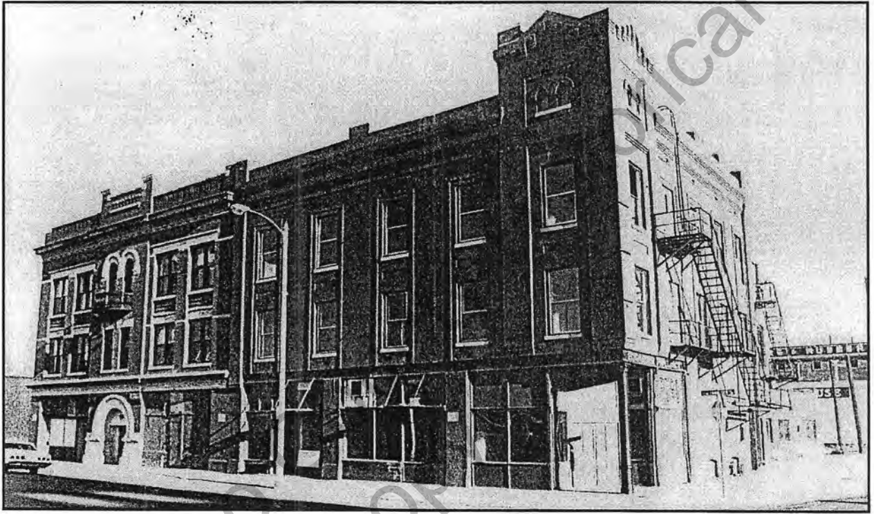
Figure 2:32. Greentree Hotel (September 1986).
