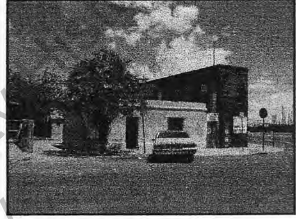
Figure 5:41. Residence-tenements in background. 426-430 Durango
