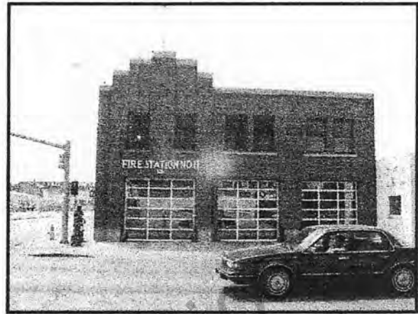
Figure 5:26. Fire Department Station #11 built in 1930. 311 Santa Fe
