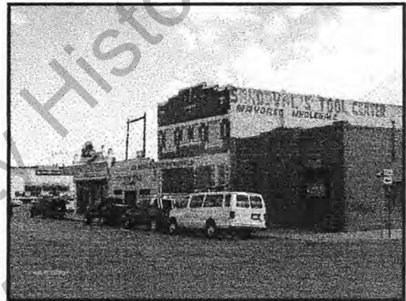
Figure 5:28. El Paso Plumbing. Previous Overall Factory. 216 W. Overland.
