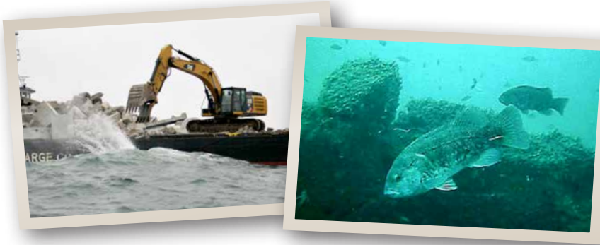
Left: An excavator deploys concrete material from a barge on the new Harwich Reef Right: Tautog photographed on the new reef in August of 2016
