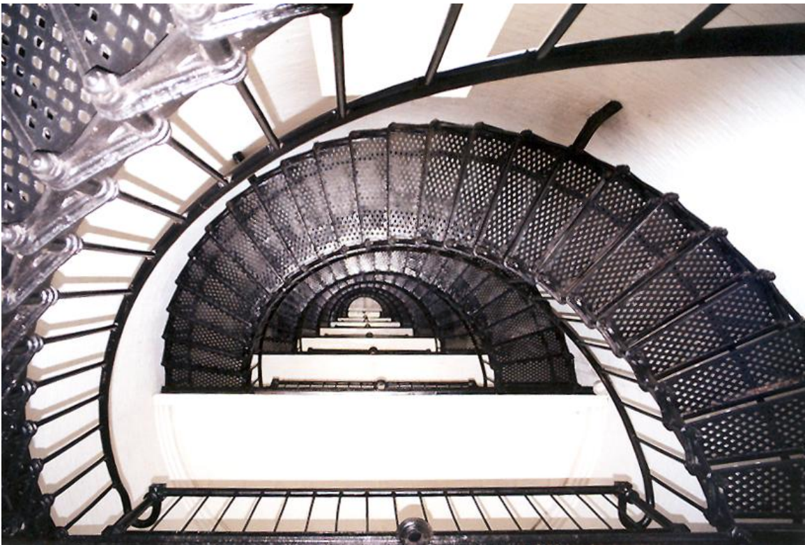
St. Augustine Light Tower Stairway
