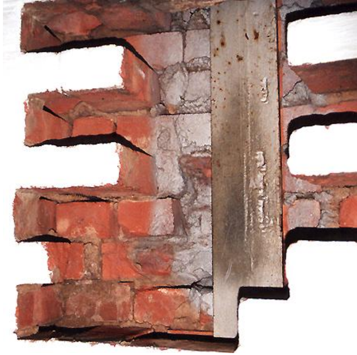
St. Augustine Light Tower Interior Wall View
