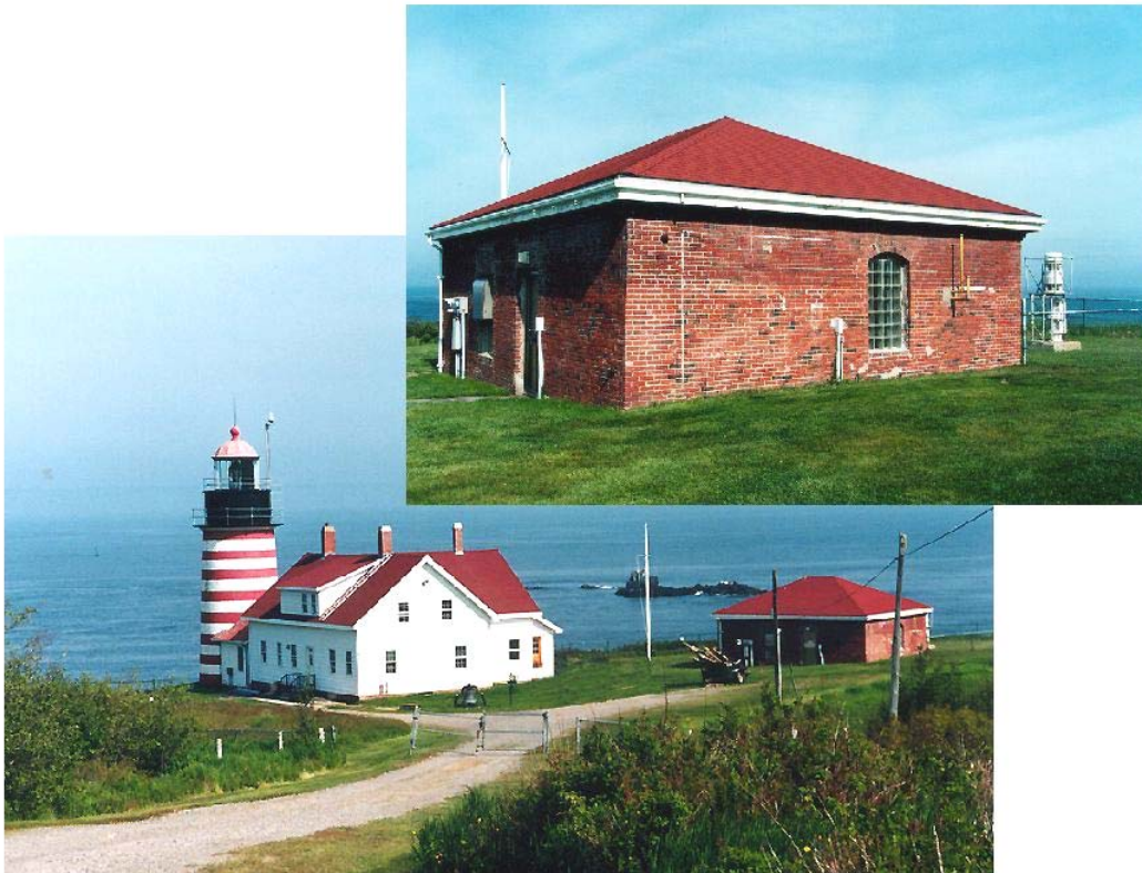
Fog Signal Building (Upper Right) and Electric Horn (Right of Building)
