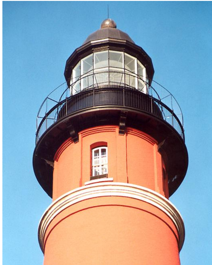
Ponce de Leon Inlet Light Lantern and Gallery Deck
