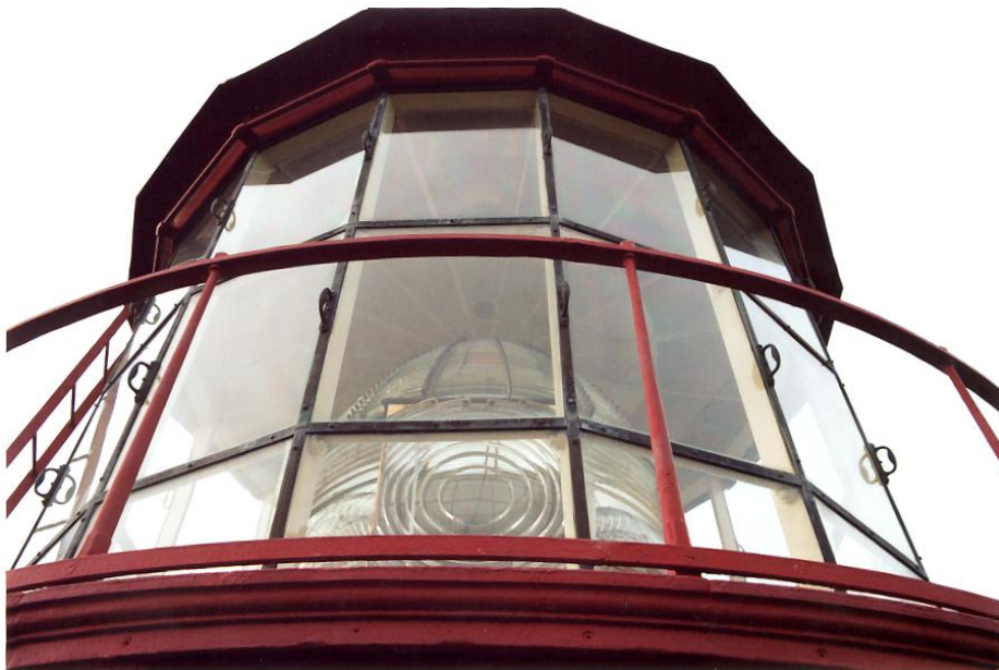
St. Augustine Light Lantern with First Order Fresnel Lens
