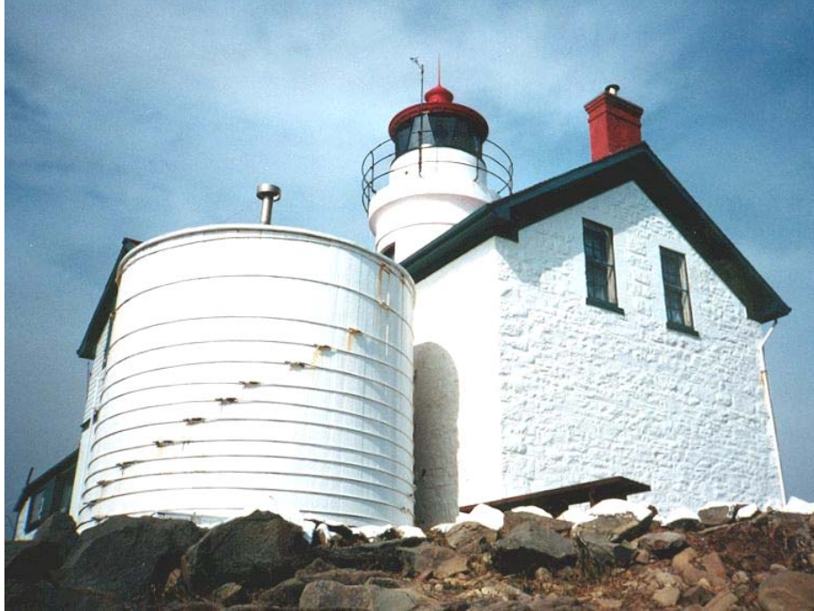
Water Holding Tank – Crescent City Light, California
