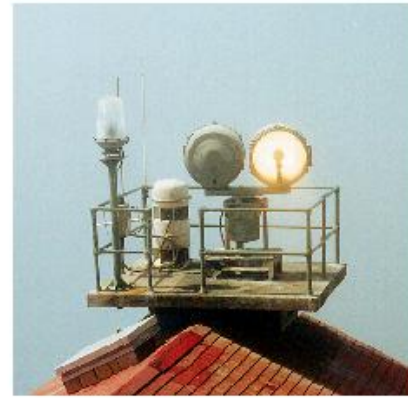
Automated Equipment Point Reyes Light Auxiliary Light, Fog Signal and Rotating Twin-Aerobeacons
