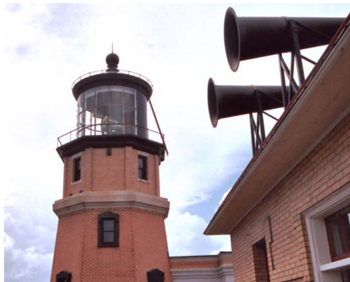
Light tower (rear) and Fog Signal Diaphones (foreground) Split Rock Light – Beaver Bay, Minnesota
