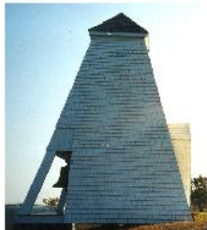
Fort Point Lighthouse Stockton Springs, Maine Fog Bell Tower
