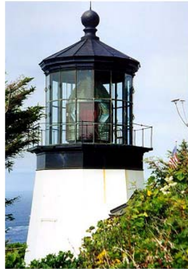
800,000 Candlepower First Order Fresnel Lens - Cape Meares, Oregon
