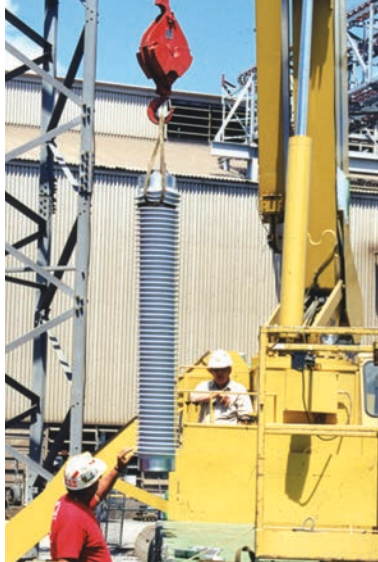
First application of hollow core composite insulators in Canada during 1990s saw them handled like porcelain.
