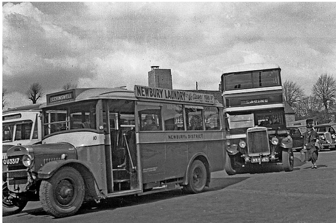
No. 10 (OU3317), was new in 1929 as a demonstrator and was acquired by Newbury & District in 1933. It was a Thornycroft A2 with Wadham 20-seat bodywork. (The Bus Archive).
