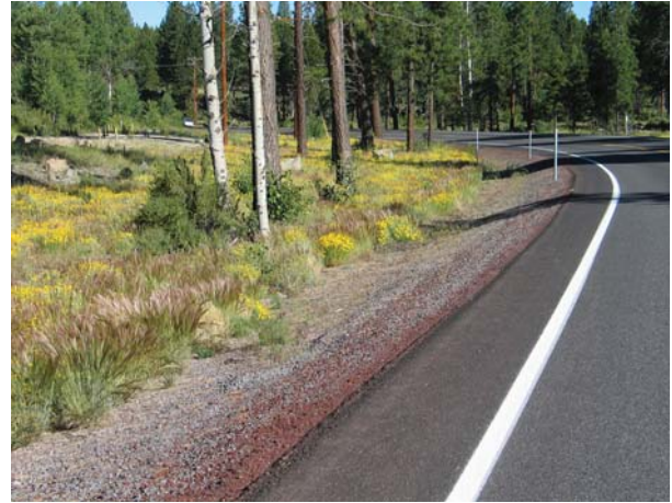
Figure 10.1.8.5. Most planting islands are designed to mimic the natural surrounding environment of the project site. In this photograph, seedlings were planted in clumps to mimic the small islands of trees that grew in this geographic area. The inter-island areas were planted with lower growing grasses, forbs, and shrubs.
