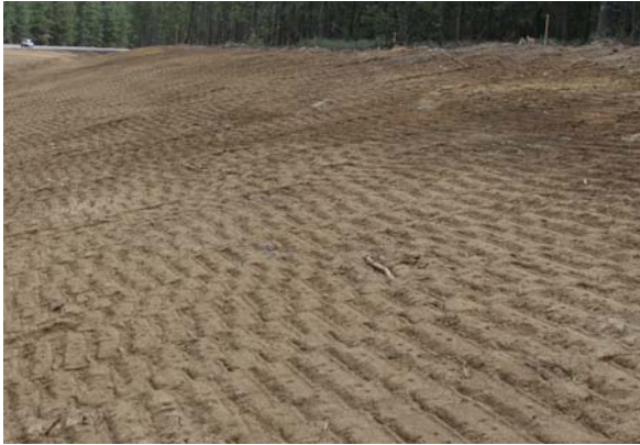
Figure 10.1.2.5. Trackwalking creates imprints on the soil surface, but will also compact surface and subsurface soils.
