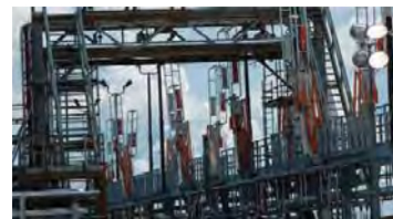
GT Omniport Unloading Area
