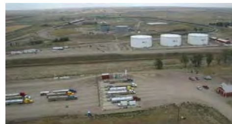
Expansion of the Inergy crude oil transfer station near Epping, N.D.
