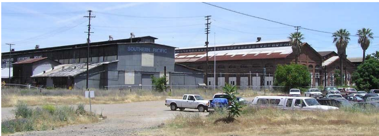
Photo 9: View of Boiler and Erecting Shop (Photo by JRP Historical Consulting, LLC; 2006)
