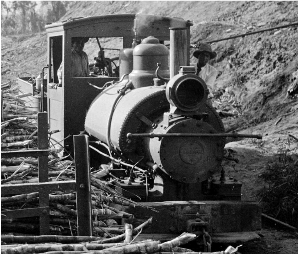
This photo supposedly showing an 0-4-0ST at Ingenio Infantas was taken by Robert H. Platt in 1930, and is from the AGSL photo archive at the University of Wisconsin Milwaukee. The front plate shows the Baldwin works number 52846 which was a 60cm gauge 0-4-0TT supplied to Peru via W. R. Grace & Co. in 1920.
