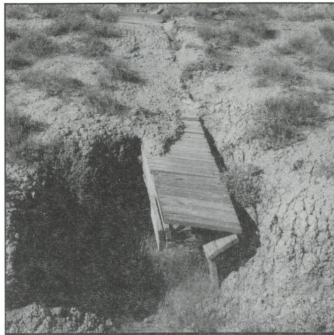
Wooden culvert on the Midland Trail on Narrow Gauge right-of-way. (Photos courtesy of author, Lloyd M. Pierson)
