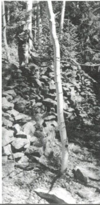
Dave Vaughn, Grand Co. Roads Dept., is seen walking along the Hepburn Road. Note the rocks stacked to reinforce a section of the road.
