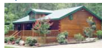
FERN GARDEN. Delightful one level 2 BR, 2 BA log cabin. Fireplace, screened porch. Outdoor fire pit. MLS #1247130. $239,000.
