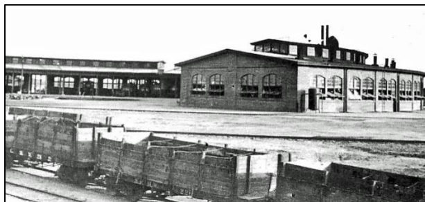
The roundhouse and shop facilities were rebuilt by 1912. (Courtesy of the Arizona Historical Society #PC180f187_4904)
