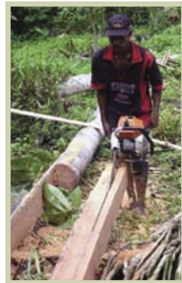
Figure 8-7. Using a chain saw on Manus Island, Papua New Guinea to mill a coconut log for structural beams. (Dan Etherington)
