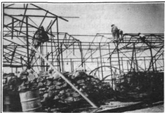
Right: The steel framework takes shape
