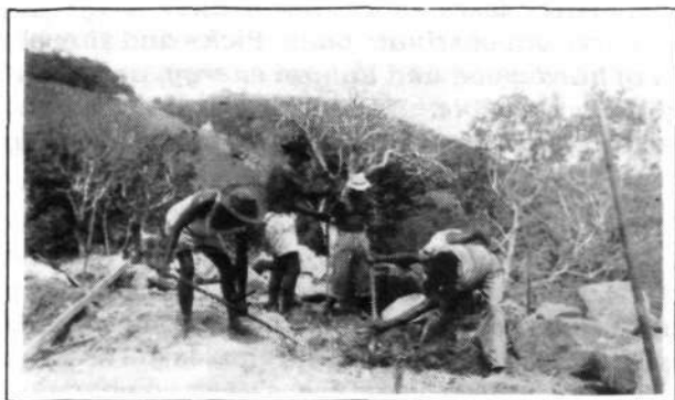
Left: Beginnings: digging the foundation trench.
