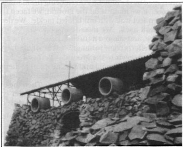
Front view (above) and side view (right) of the new church, showing windows in position and the stone work gradually enclosing them
