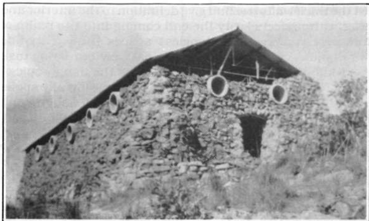
Front view (above) and side view (right) of the new church, showing windows in position and the stone work gradually enclosing them
