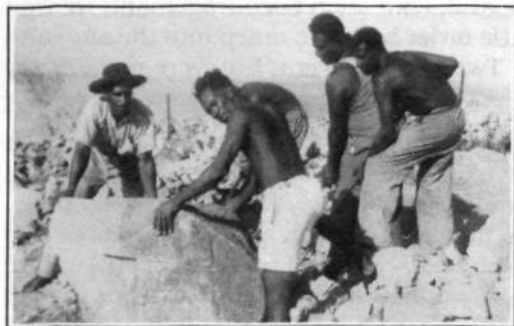
Left: No. 1 boulder goes into the foundations
