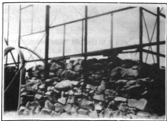
Left: The interlacing of the stones with the steel work of the army huts
