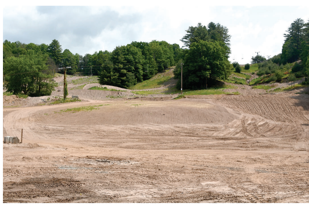
Work has already begun on reshaping the ski hill, repairing it from erosion, which new owner, Michael Taylor, said is an unending problem.
