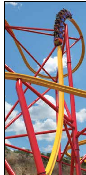
Six Flags Fiesta Texas will debut Wonder Woman Golden Lasso in the spring. It will be the first coaster to feature Rocky Mountain Construction's Raptor Track and will include inversions, an overbanked turn and a 90-degree first drop (right). Riders will be positioned in new trains that sport a single-file configuration. COURTESY SIX FLAGS FIESTA TEXAS
