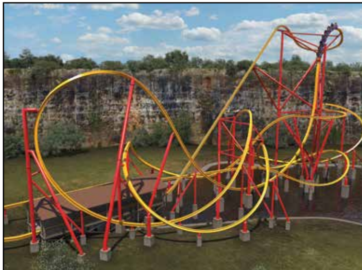
Six Flags Fiesta Texas will debut Wonder Woman Golden Lasso in the spring. It will be the first coaster to feature Rocky Mountain Construction's Raptor Track and will include inversions, an overbanked turn and a 90-degree first drop (right). Riders will be positioned in new trains that sport a single-file configuration. COURTESY SIX FLAGS FIESTA TEXAS
