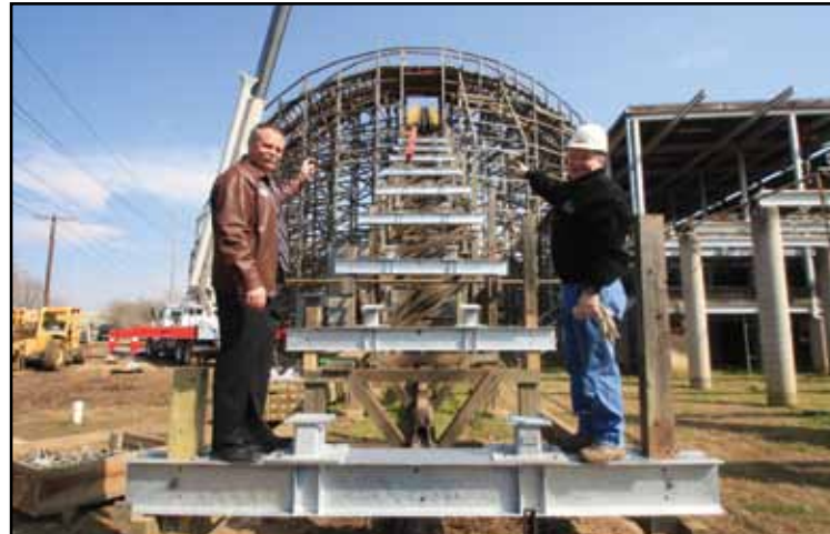
Six Flags Over Texas Park President Steve Martindale, left, and Rocky Mountain Construction President, Fred Grubb, point to the new I-Box track design (shown at right) currently being installed on the park's Texas Giant. The ride will reopen in 2011.
