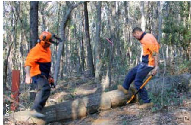
Figure 6.33: Workers clear and widen a section of the Bundian Way, the first Aboriginal pathway to be listed on the New South Wales State Heritage Register
