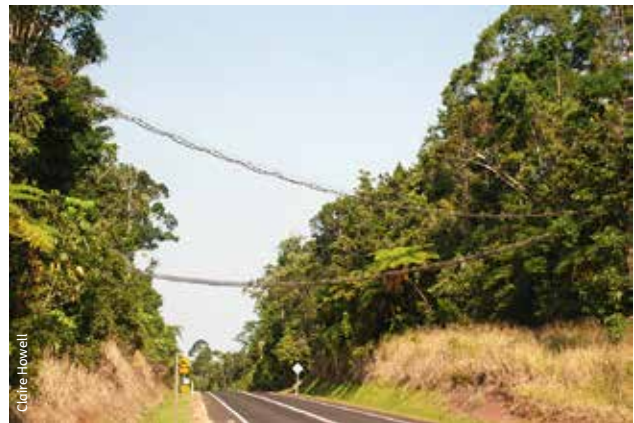
Possum bridge to allow animals to move between forest fragments and maintain connectivity of populations.
