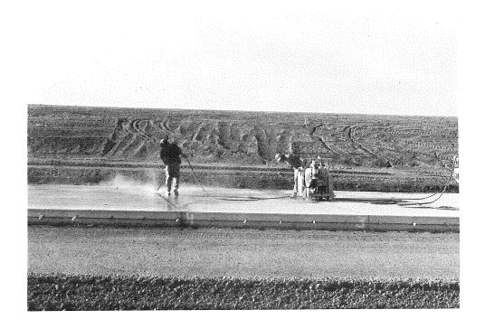
Figure 6 - Water Jetting and Dry Sawing Transverse Joints
