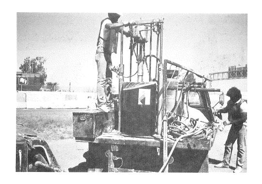
Figure 14 - Pumping Equipment for Installation of Sealants
