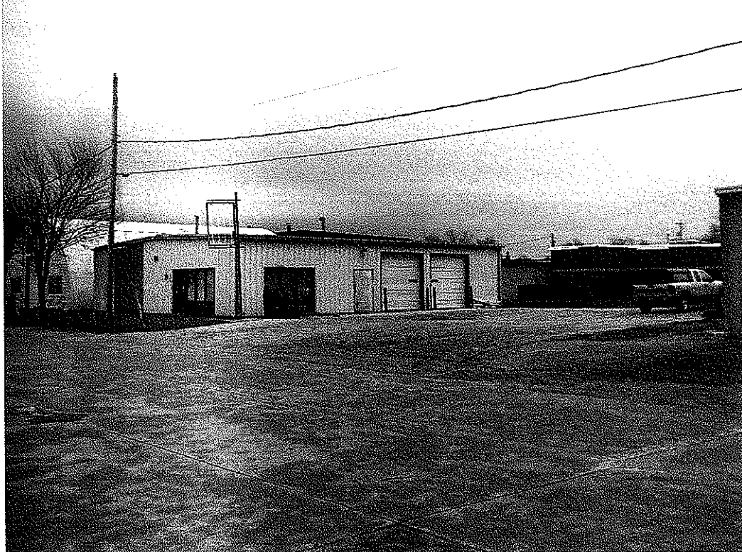
Photo #1: Looking southeast.
