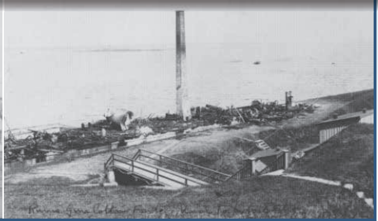
Before and after pictures of the gun cotton factory at the Naval Torpedo Station reveal the effects of a disastrous explosion on July 3, 1893, that killed three men and injured 10 others. The explosion was found to be caused by a fire that originated in the "picked-cotton room" where a machine picked apart raw English cotton. A foreign object in the cotton struck the teeth of the picker resulting in a spark that ignited the cotton. (Photo source: "A Century of Progress," p. 33)
