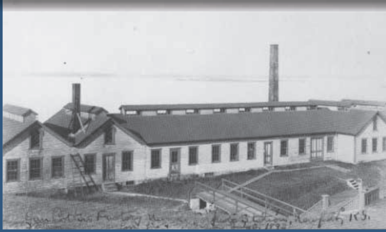
Before and after pictures of the gun cotton factory at the Naval Torpedo Station reveal the effects of a disastrous explosion on July 3, 1893, that killed three men and injured 10 others. The explosion was found to be caused by a fire that originated in the "picked-cotton room" where a machine picked apart raw English cotton. A foreign object in the cotton struck the teeth of the picker resulting in a spark that ignited the cotton. (Photo source: "A Century of Progress," p. 33)
