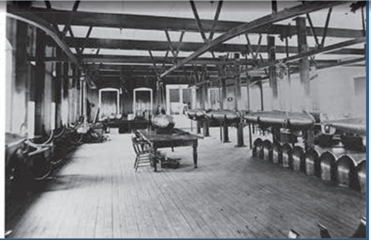
This Whitehead Mark 5 torpedo (left photo), the first torpedo to be purchased by the U.S. Navy, was fitted with a net cutter in this 1908 photo taken at the Naval Torpedo Station. (Source: Naval History and Heritage Command) Whitehead torpedoes are shown in the Torpedo Overhaul Shop (right photo) at the Naval Torpedo Station on Goat Island in 1908. Note the overhead track and simple crane mechanism (block and tackle) used to transport the torpedo to the work station in the center of the room consisting of a wood table and chair. (Photos courtesy Naval War College Museum)
