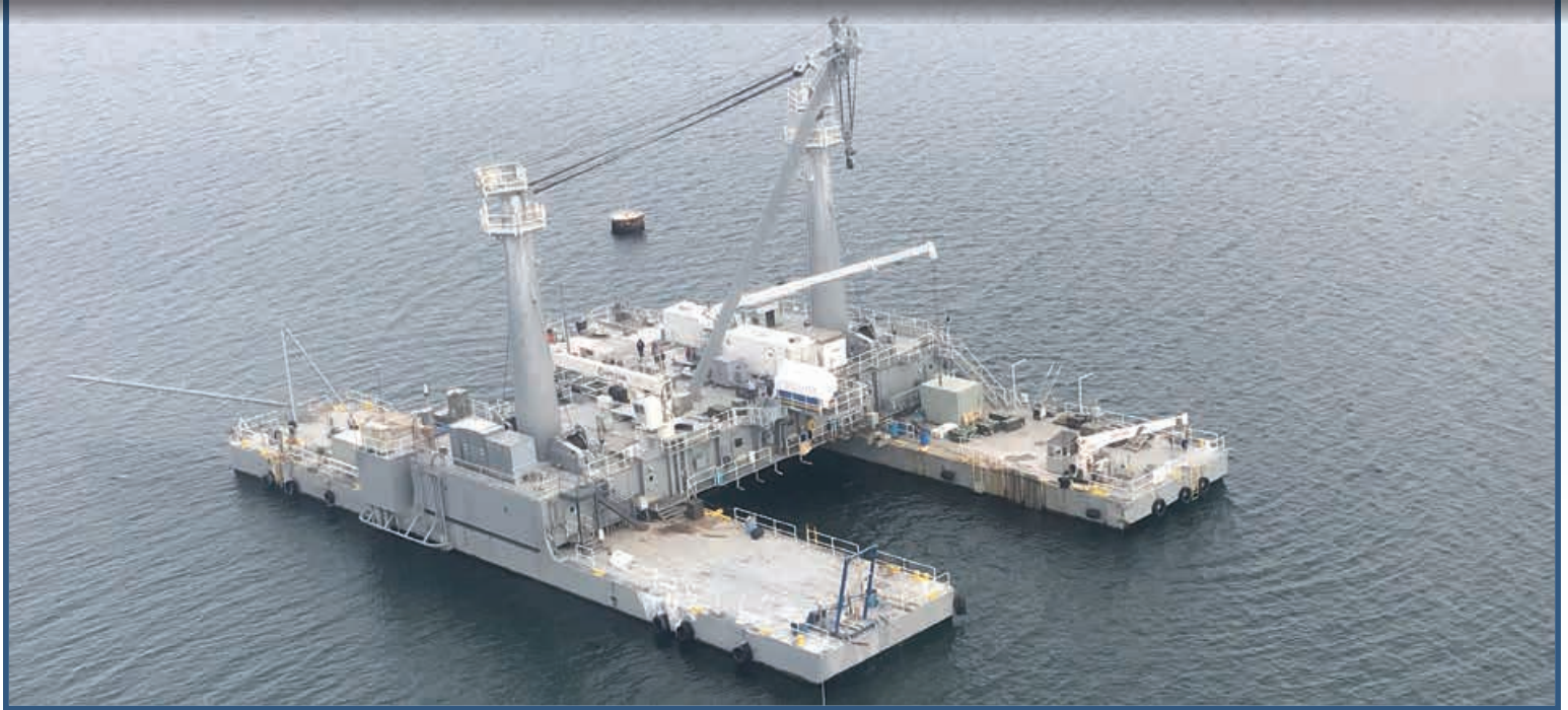
The Systems Measurement Platform at NUWC Division Newport's Seneca Lake Sonar Test Facility, located in Dresden, New York, is a massive catamaran-type platform with a 220-ton crane built into its superstructure. The Navy's primary underwater test facility, it was established for evaluating active and passive acoustic devices from a single element to a full sonar system. (U.S. Navy photo)
