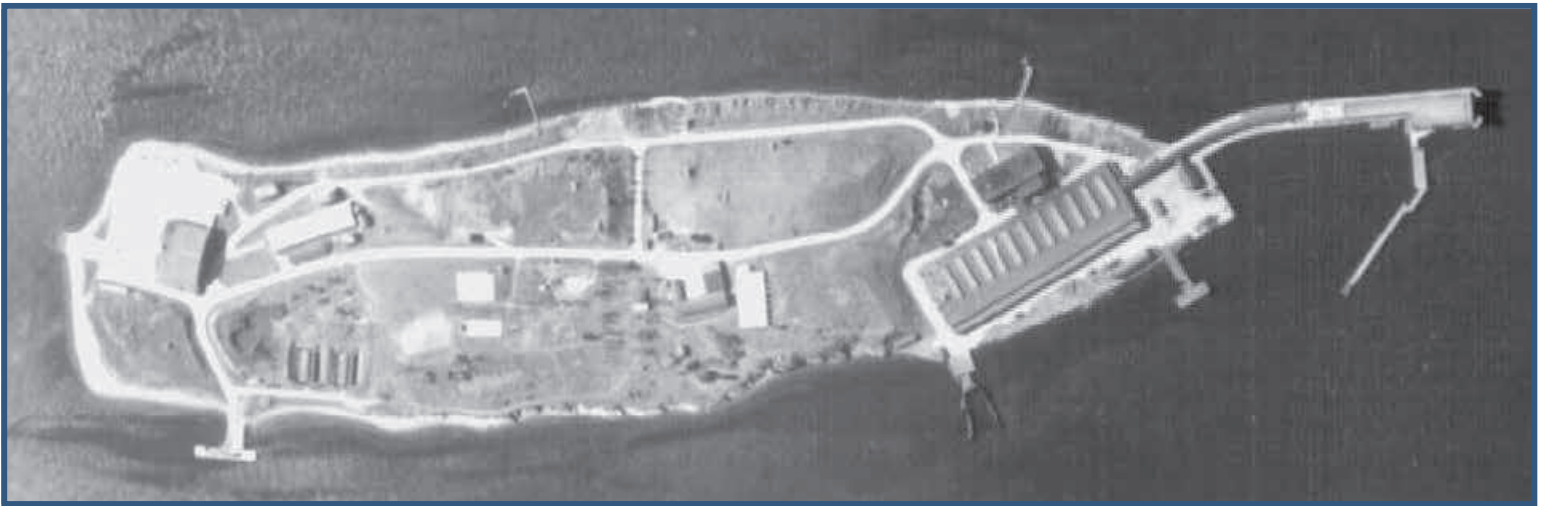
In 1909, the federal government purchased a portion of Gould Island, a 56-acre tract located in the middle of Narragansett Bay. In this 1951 aerial view (from the R.I. Geological Information Services at the University of Rhode Island), the torpedo test station is visible at the north end of the island. The seaplane facility at the south end appears to have been closed, as there are no aircraft visible on the island.
