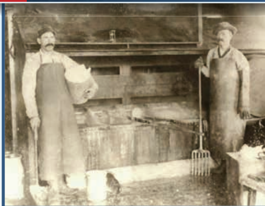
The steps to process guncotton included the nitration process (left photo), known as the nitrate bath. Prior to 1900, raw English cotton was picked apart by a machine (center photo) then washed in nitrate and taken to a separate building where the cotton was reduced to a pulp and solidified. To create the torpedo warheads, a saw (right photo) was used to cut the solidified pulp into the necessary dimensions. (Courtesy of "A Century of Progress")
