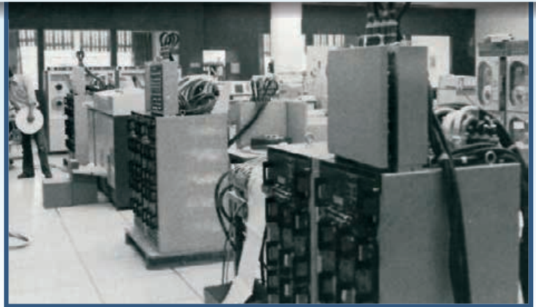
The Submarine Integrated Attached Center in Newport, as shown in 1975, supported the advanced combat systems research and development program.
