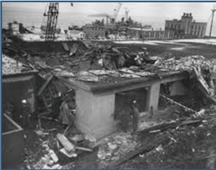
On Tuesday, April 26, 1955, an explosion occurred at approximately 11 a.m. in a dynamometer test room in Building 115. The blast is believed to have resulted from a high-pressure airline rupture while testing a high-energy monopropellant fuel, called normal propyl nitrate, in a modified Mark 16 Mod 3 torpedo.
