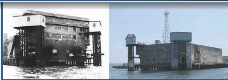
The Firing Pier on the north end of Gould Island (left photo, undated) and in 2006 (right photo). In 2000 and 2001, the upper two floors of the Firing Pier were torn down. (Source, left photo Naval War College; right photo, George DiGregorio in 2006)
