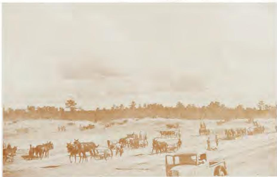
*Scores of mule teams and hired labor clear the route of the ship canal; October 11, 1935. Courtesy Corps of Engineers.*
