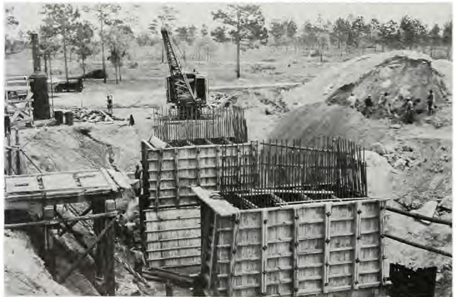
*Workers are about ready to pour concrete as work on ship canal progresses in late 1935. Courtesy Corps of Engineers.*
