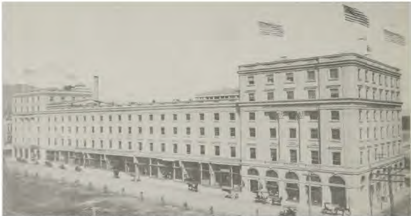
The Alexander Young Building, Bishop Street, Honolulu, where the Honolulu Engineer District (HED) maintained its offices from 1905 to 1907 and again in 1941.
