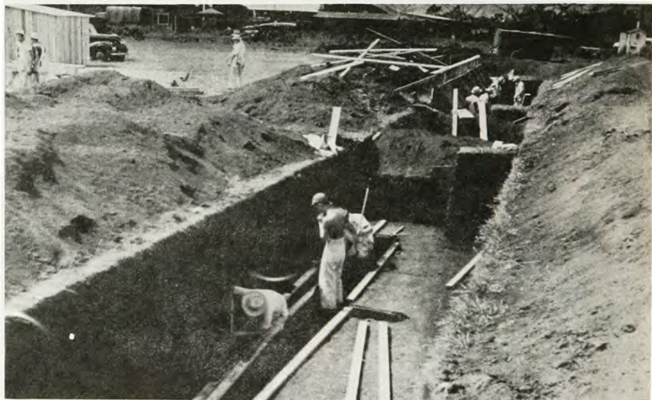
Excavation for a bombproof shelter on Oahu, 1942.
