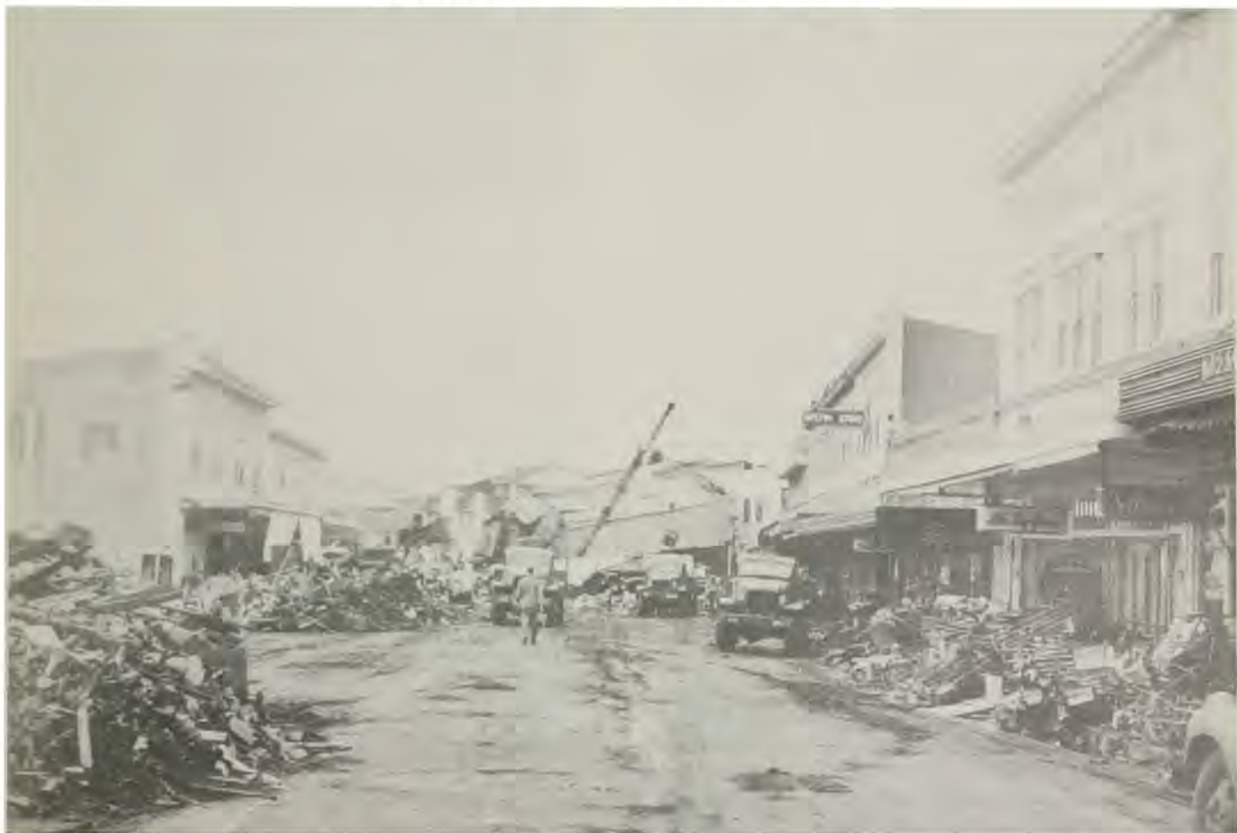
Main street of Hilo, Hawaii, after tsunami of 1 April 1946.
