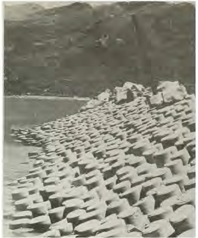
Tribars placed on the breakwater at Nawiliwili Harbor, Kauai.
