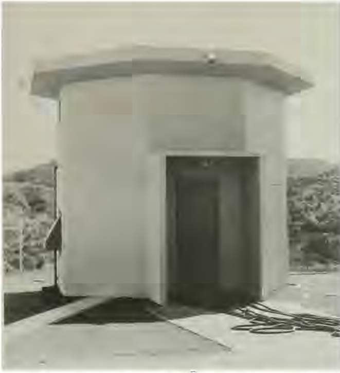
Radome support structure, Kaena Point, Oahu, 1964.
