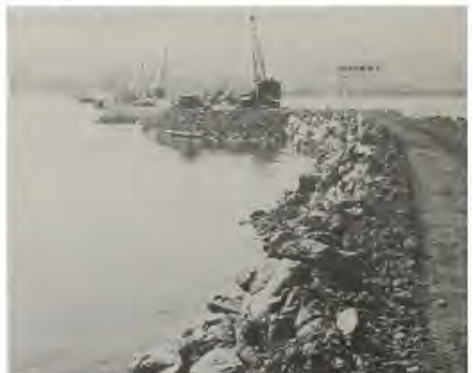
View of Hilo Harbor breakwater showing breaks in barrier August 1947.
