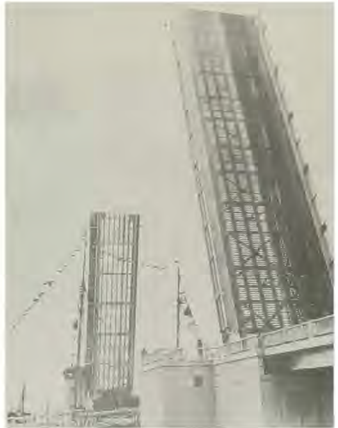
Slattery Bridge, over Kalihi Channel, Honolulu Harbor.
