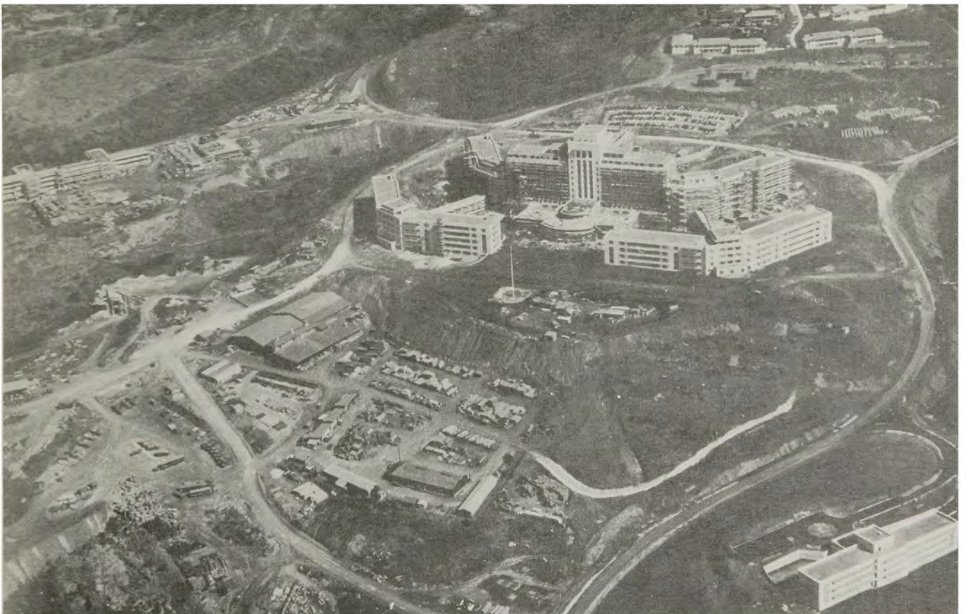
Aerial view of Tripler Hospital during final stages of construction in 1948.
