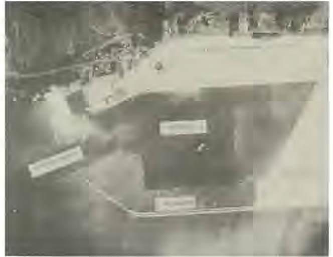
Aerial view of Kawaihae Harbor, Hawaii, January 1959.
