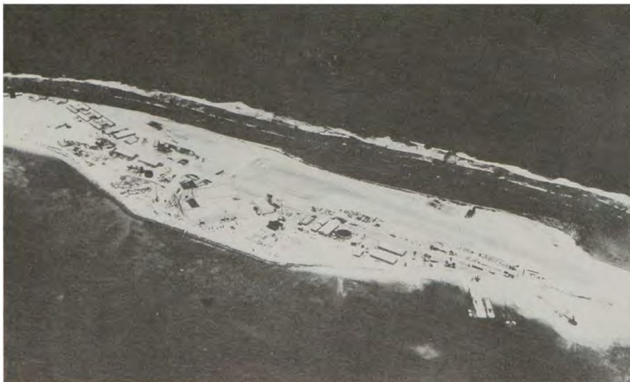
Meck Island in 1967, after clearing, grading, fill placement, and partial construction of Nike-X facilities.
