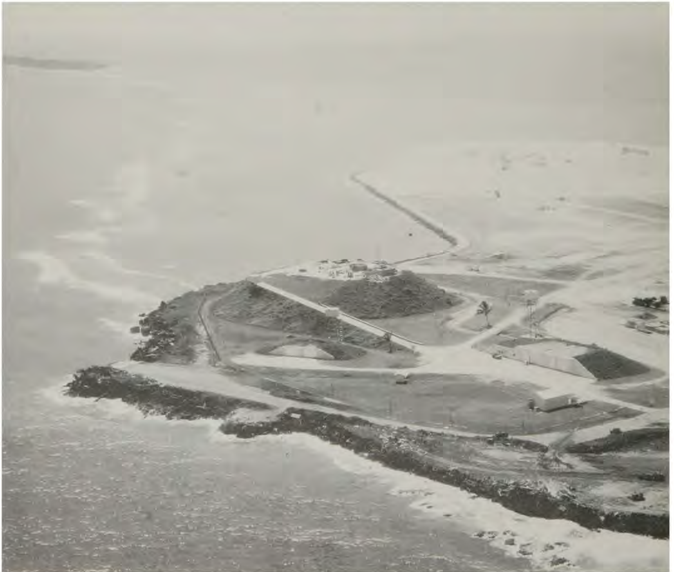
Launch facilities constructed for Nike-Zeus on the western end of Kwajalein.
