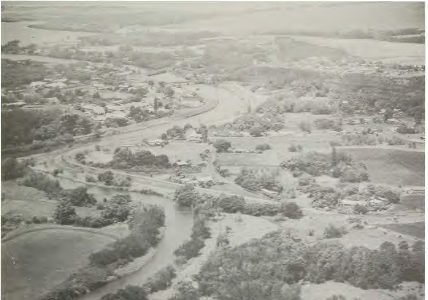
Completed flood control improvements at Hanapepe River, Kauai, looking south.
