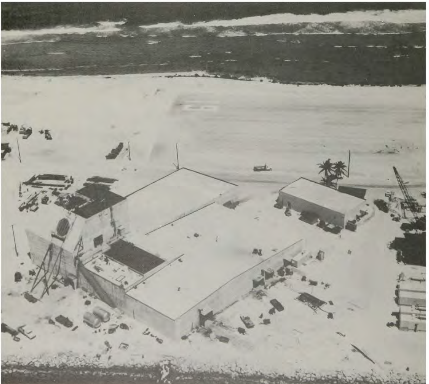
Construction of Meck Island Control Building, September 1967.
