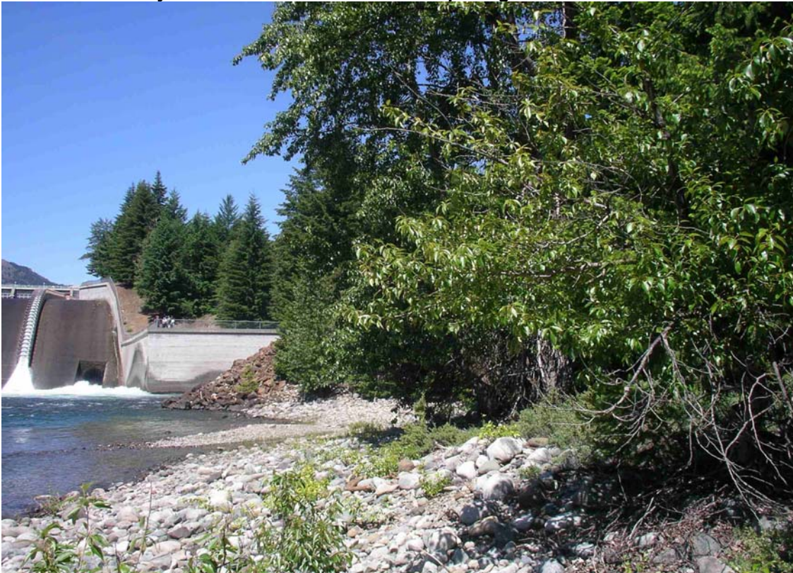
Figure 4-2. Riparian vegetation removed for construction of the adult collection facility. This figure shows the Alternative 2 location of the adult collection facility.
