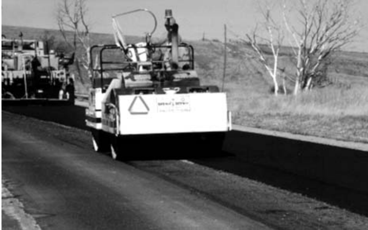
Figure 16-8: Finishing rolling
