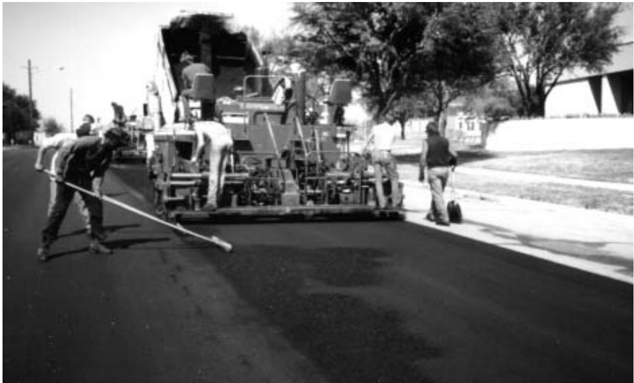
Figure 6-21: Recycled mix and integral overlay ready for compaction
