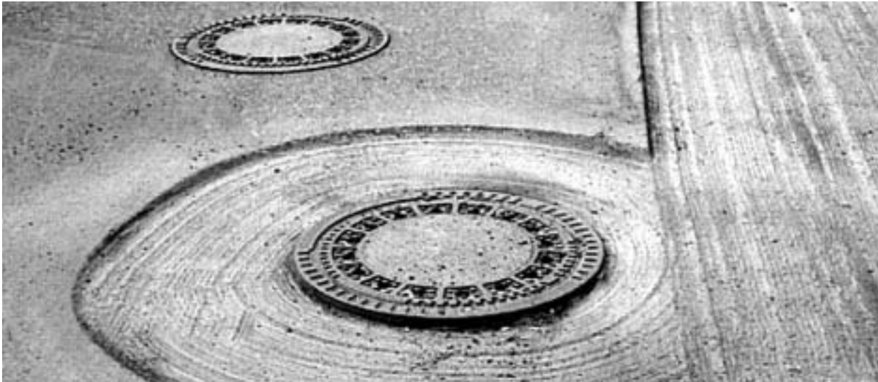
Figure 8-9: Milling around street castings
