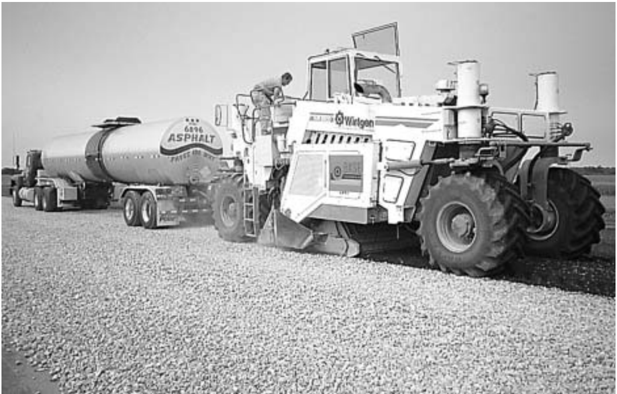
Figure 1-16: FDR reclaimer and stabilizing additive tanker
