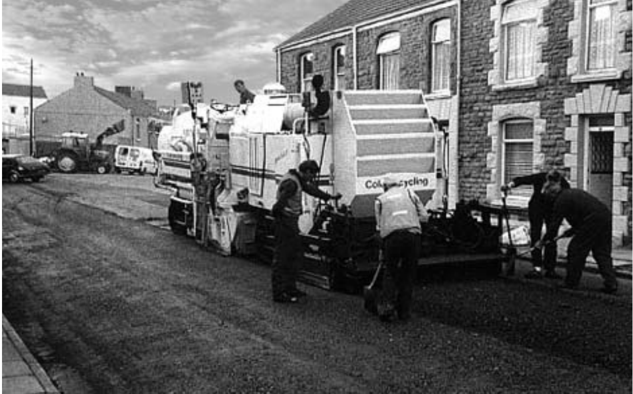
Figure 1-18: Single unit CIR train
