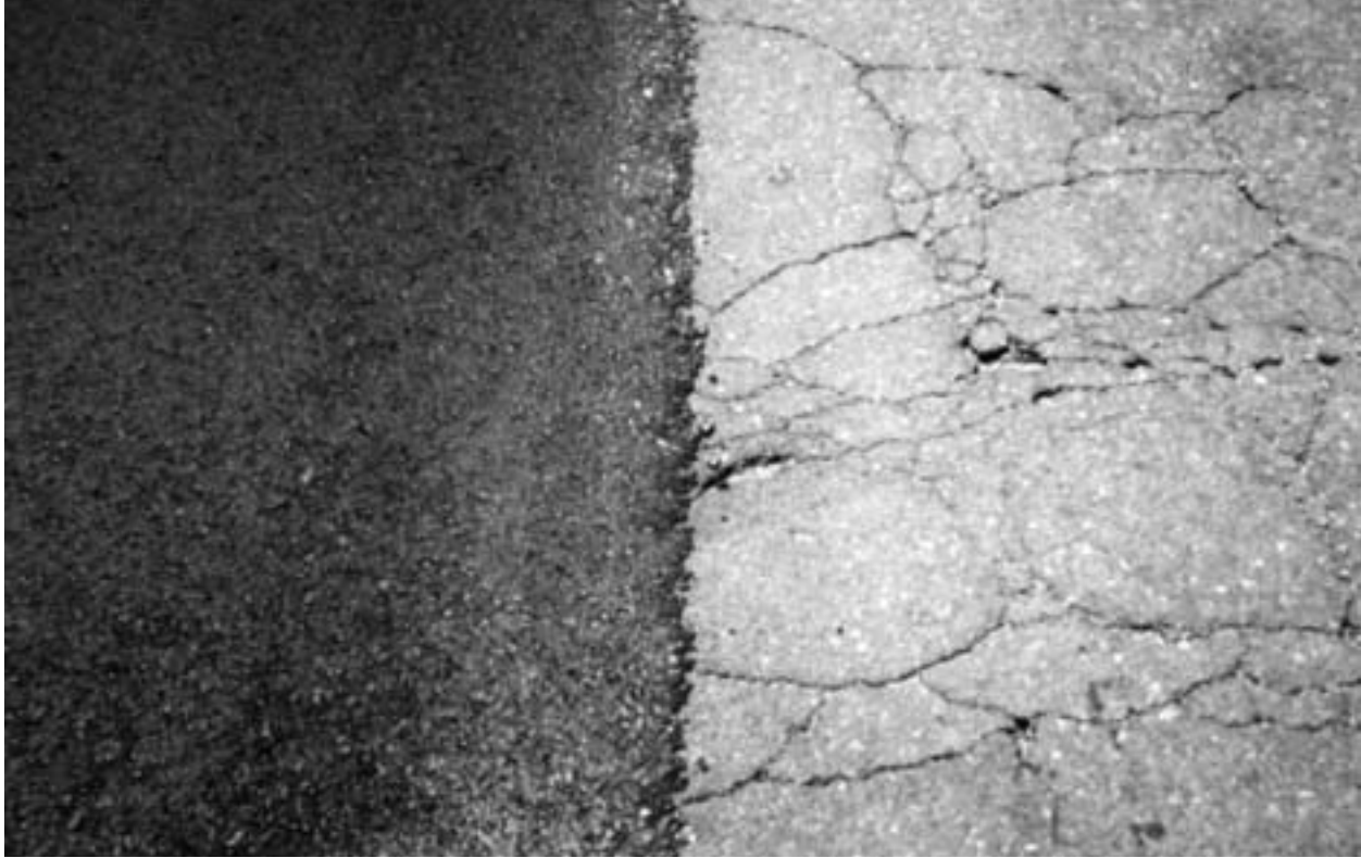
Figure 6-10: Surface Recycling before and after
