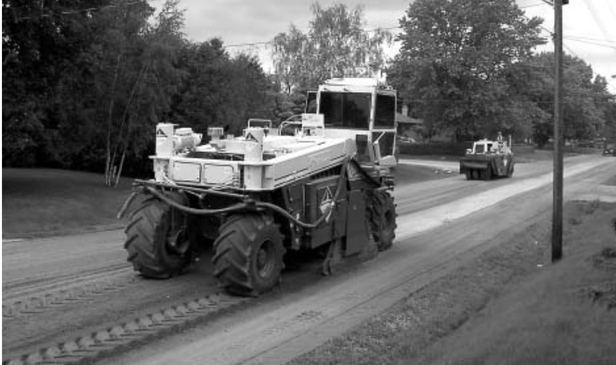
Figure 12-7: Reclaiming operation
