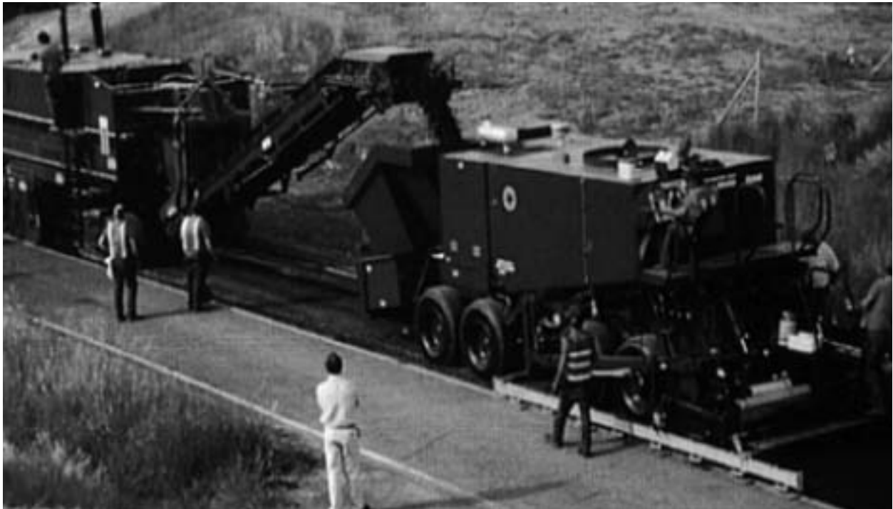
Figure 1-19: Two-unit CIR train
