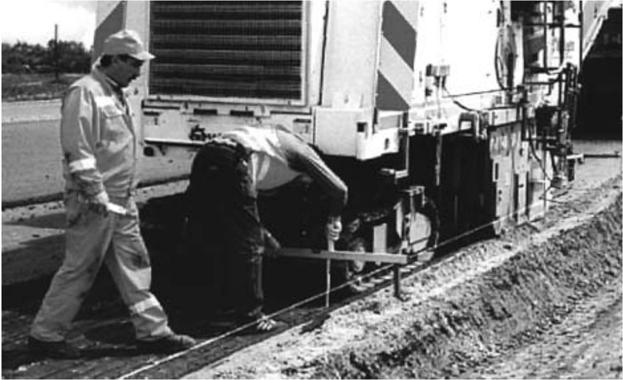
Figure 8-7: Transducing sensor and stringline for control of the cutting drum
