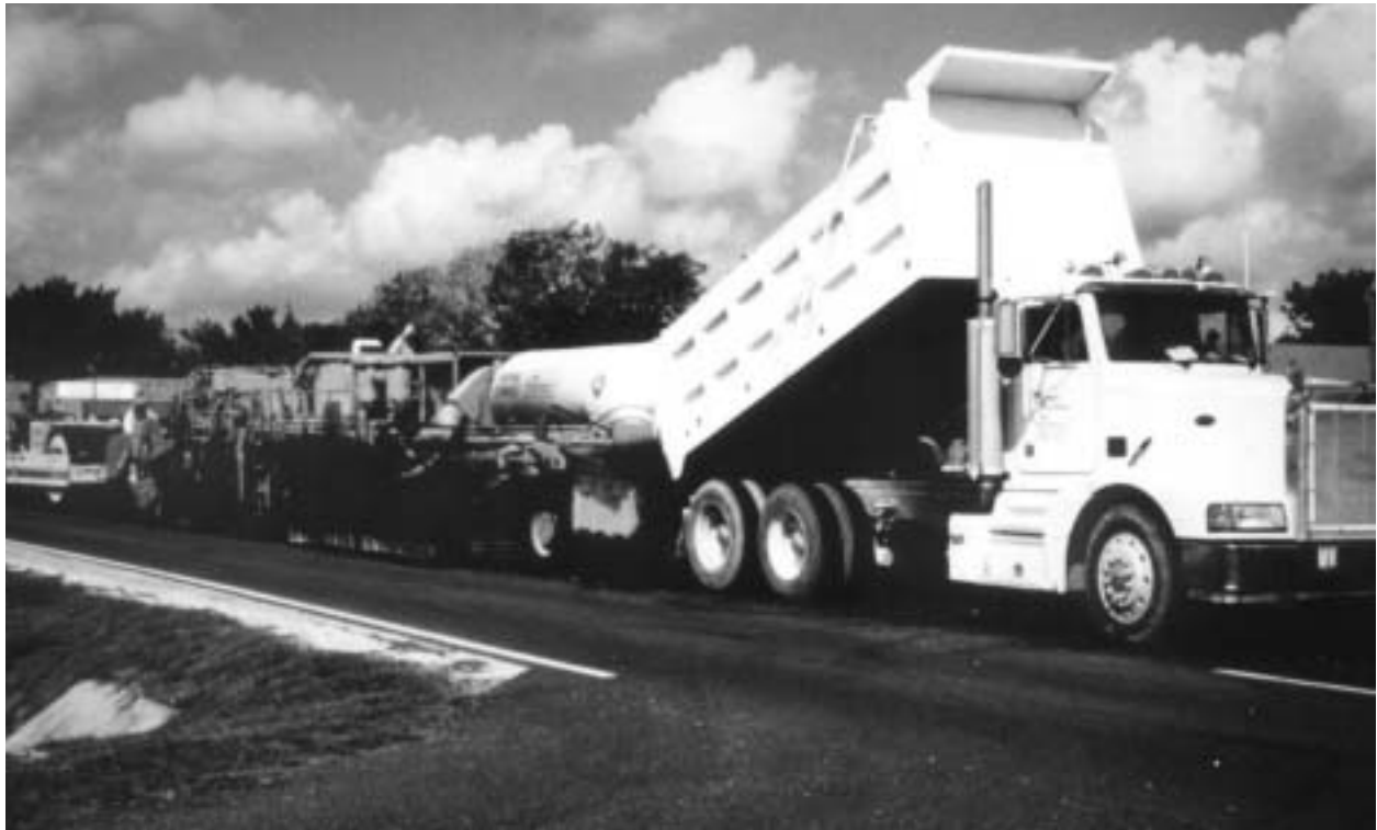
Figure 6-20: Repaving c/w haul truck for integral overlay
