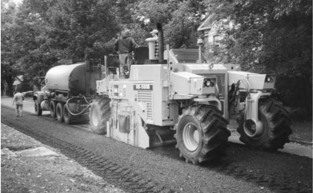
Figure 11-3: Asphalt emulsion stabilization in urban setting
