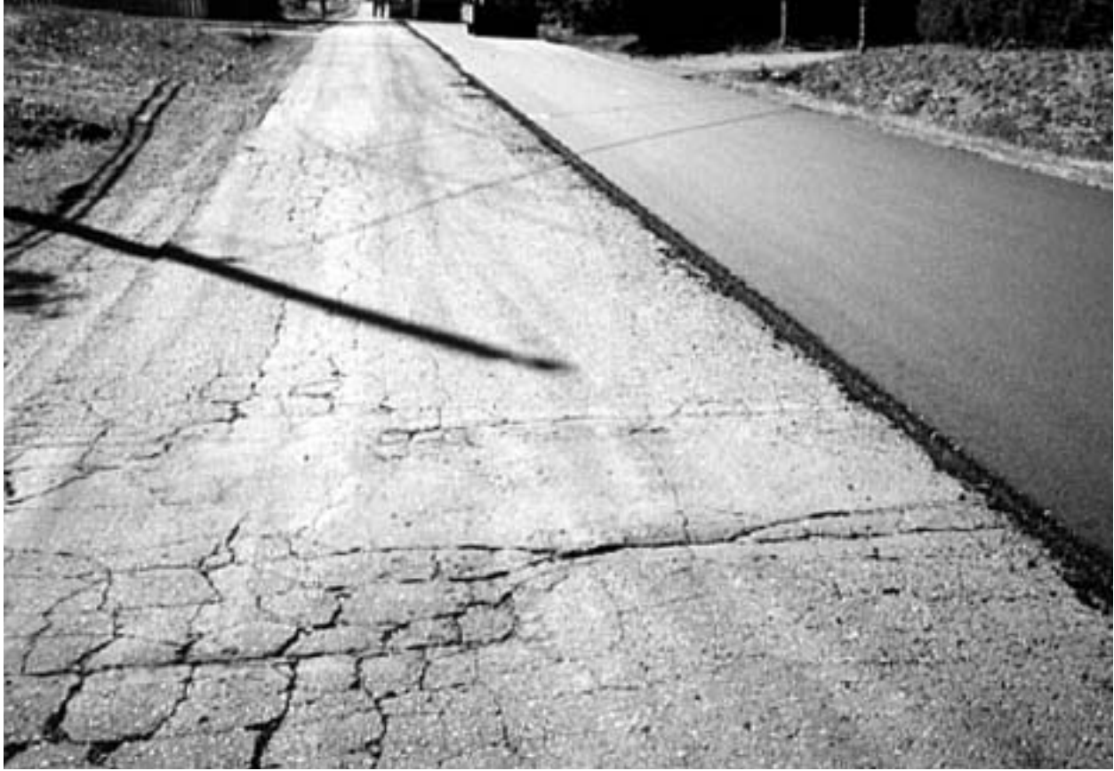
Figure 6-23: HIR Repave before and after
