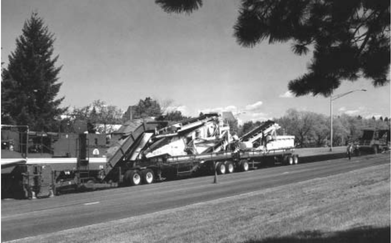
Figure 16-3: Cold In-Place Recycling Arterial City Streets
