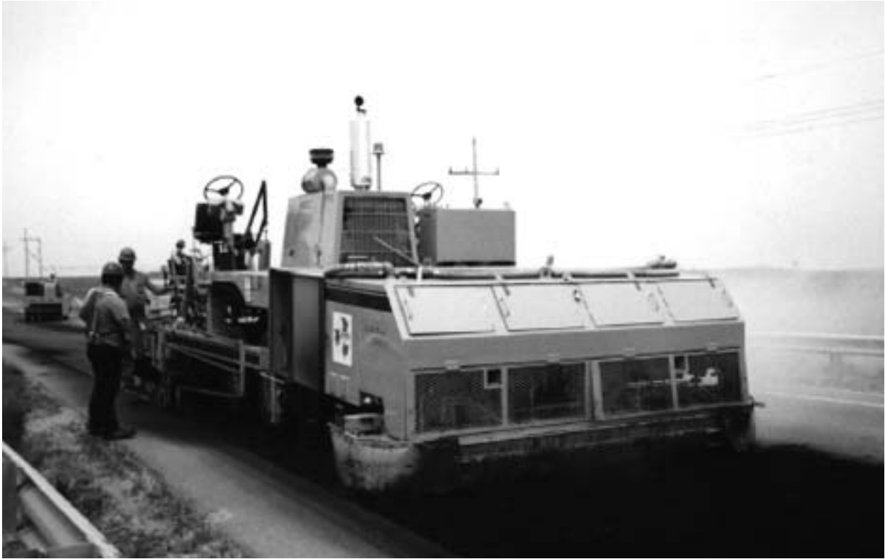
Figure 6-5: Recycling agent addition, mixing, and paving unit
