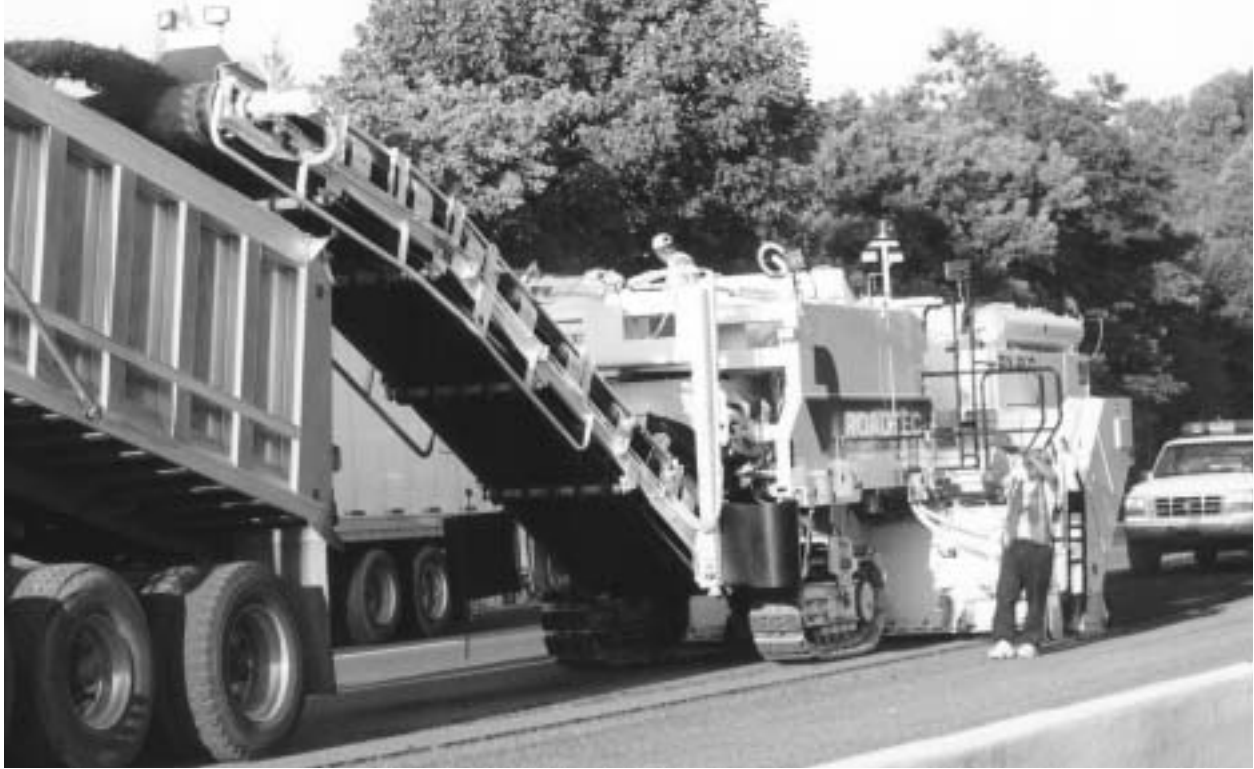
Figure 8-6: Front loading milling machine
