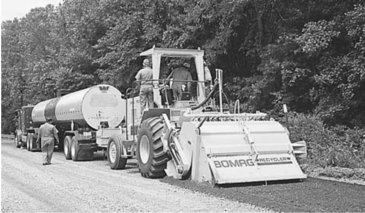
Figure 12-9: Stabilizing Agent Addition
