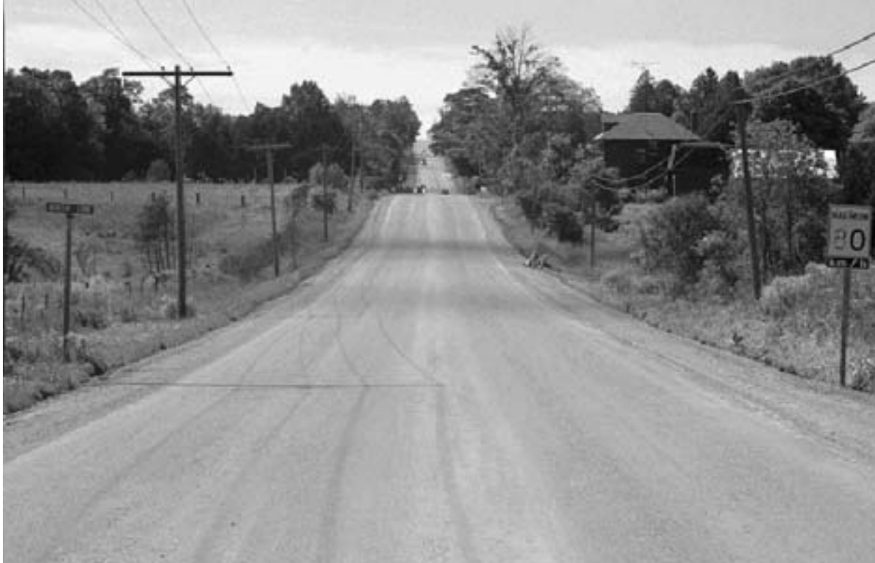
Figure 12-10: Bituminous stabilization mat prior to placement of wearing surface.
