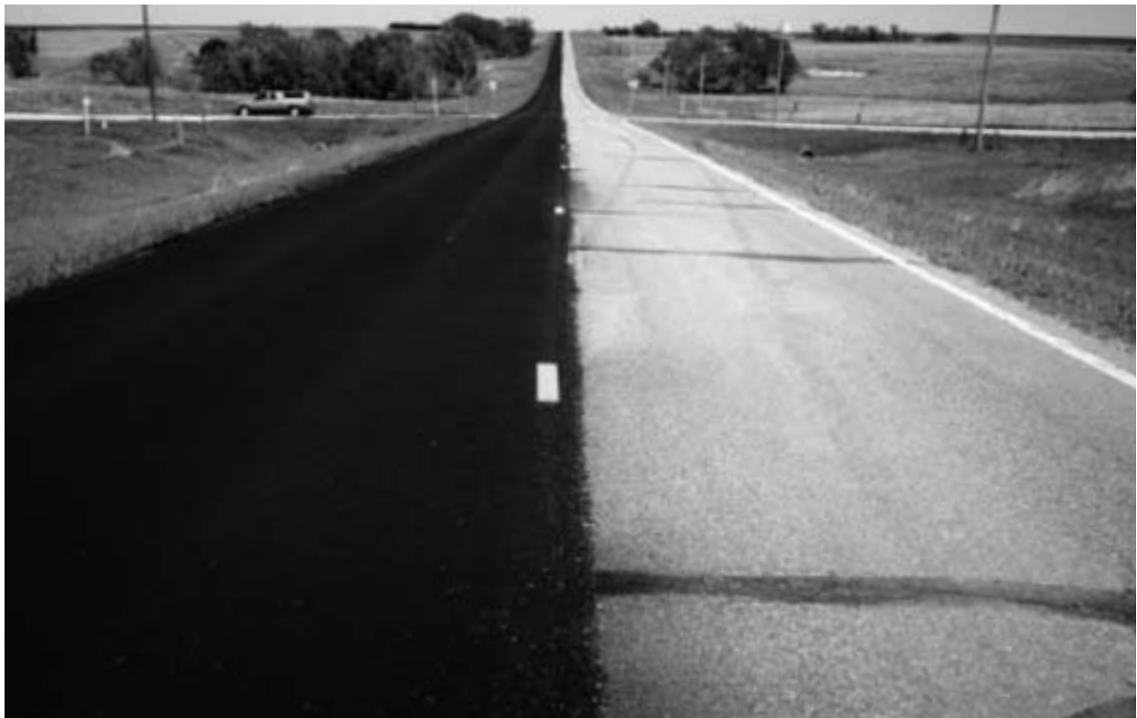
Figure 6-9: Surface Recycling before and after
