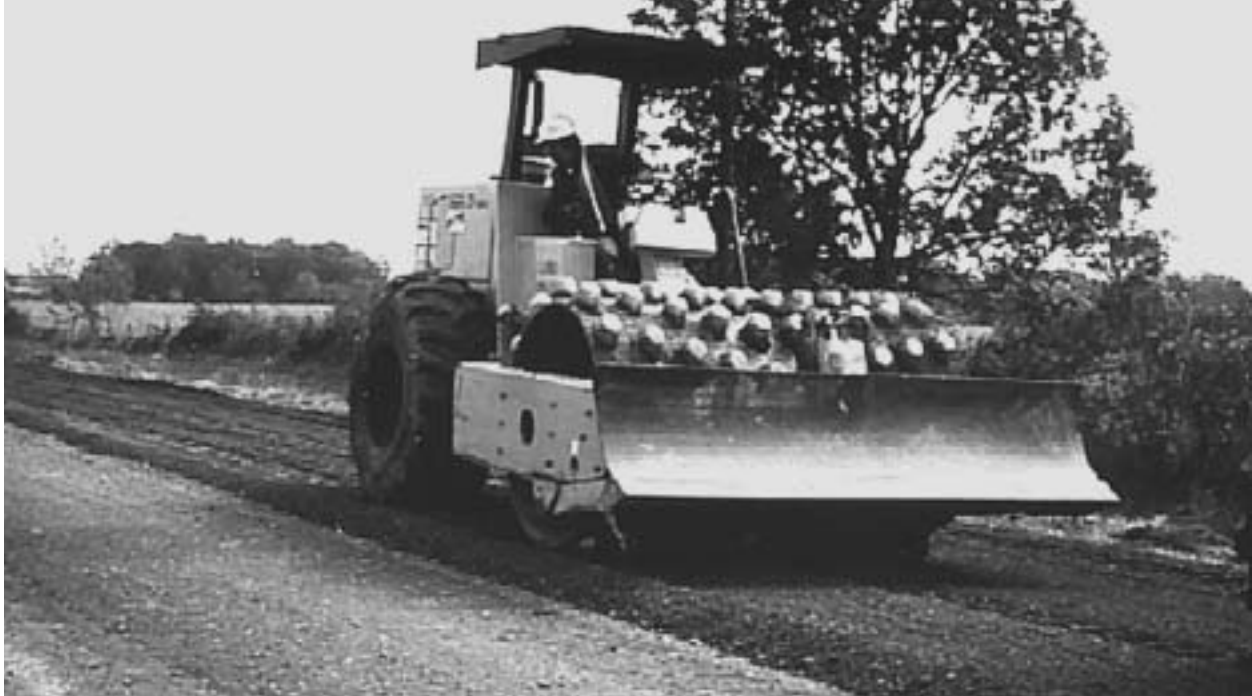
Figure 12-6: Compaction of FDR mix
