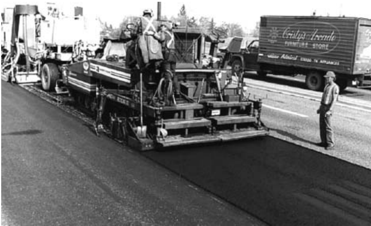
Figure 6-17: Conventional HMA paver placing recycled mix
