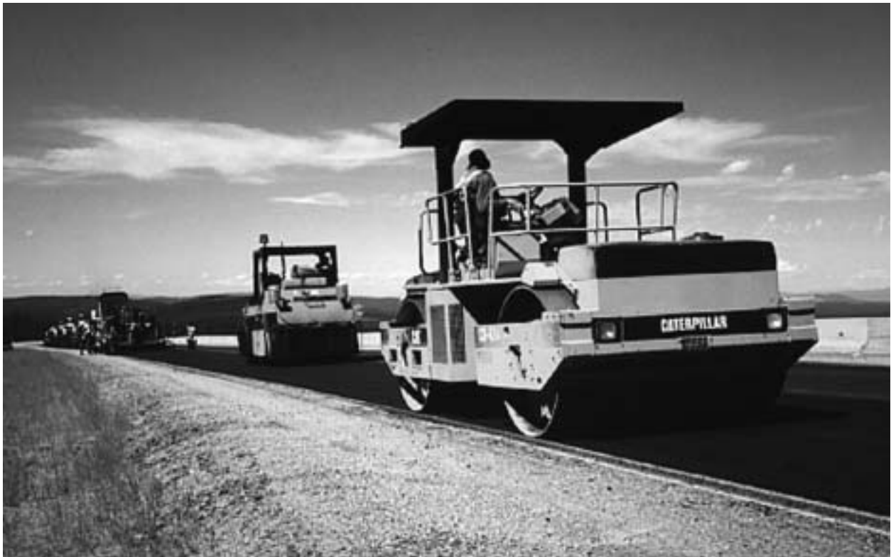
Figure 6-19: Compaction of recycled mix
