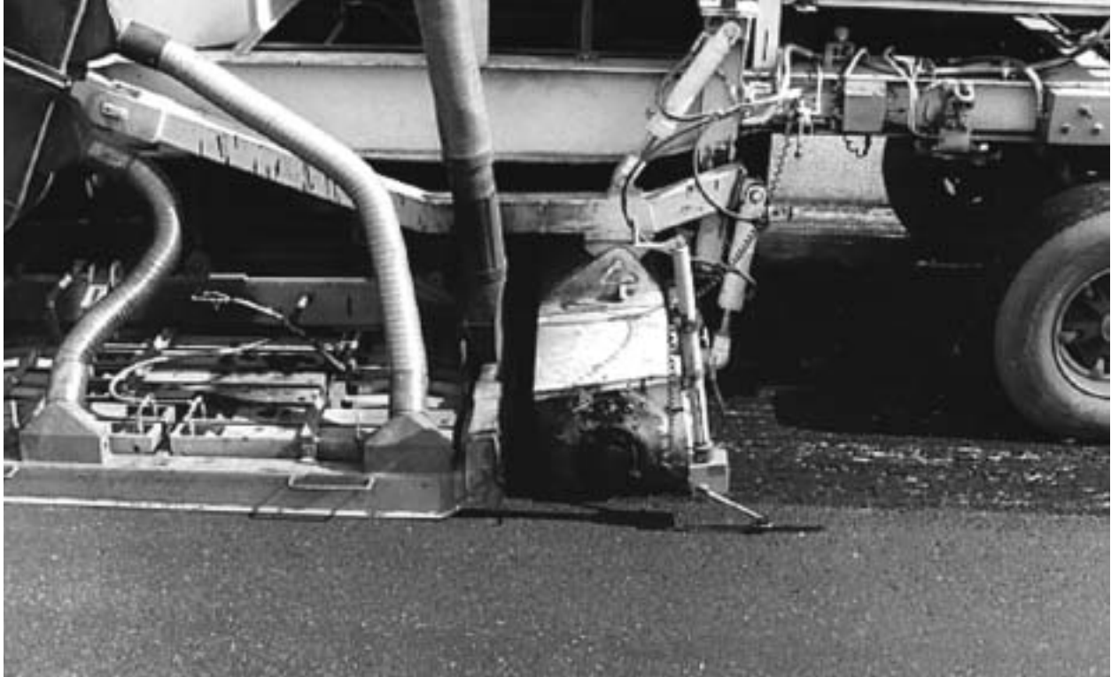
Figure 6-13: Hot milling drum and matching shoe
