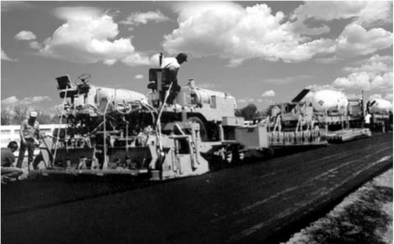
Figure 1-9: Recycled mix placement
