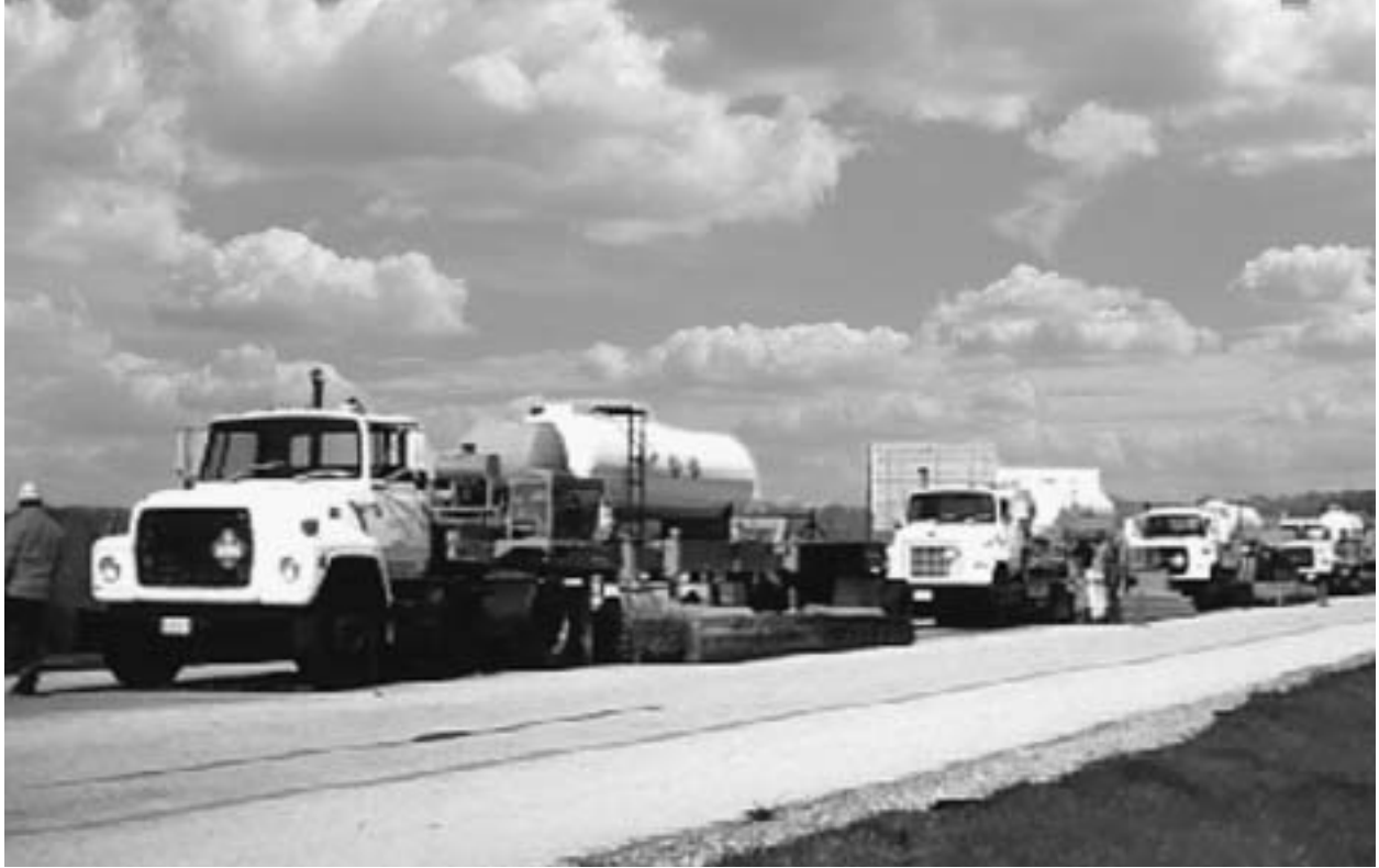
Figure 6-1: Surface Recycling preheaters
