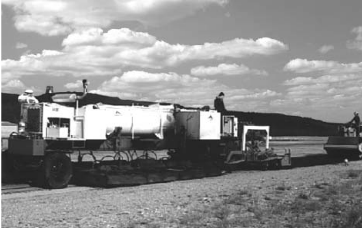
Figure 6-7: Free floating screed on scarification unit
