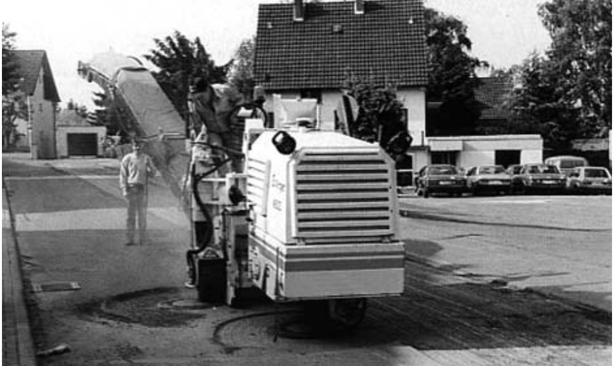
Figure 8-1: Mini cold planer working around a manhole
