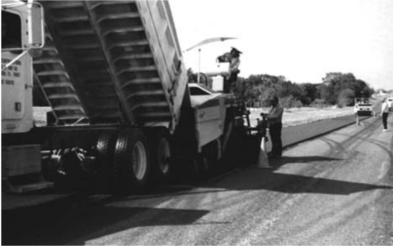
Figure 1-24: CCPR mix placement
