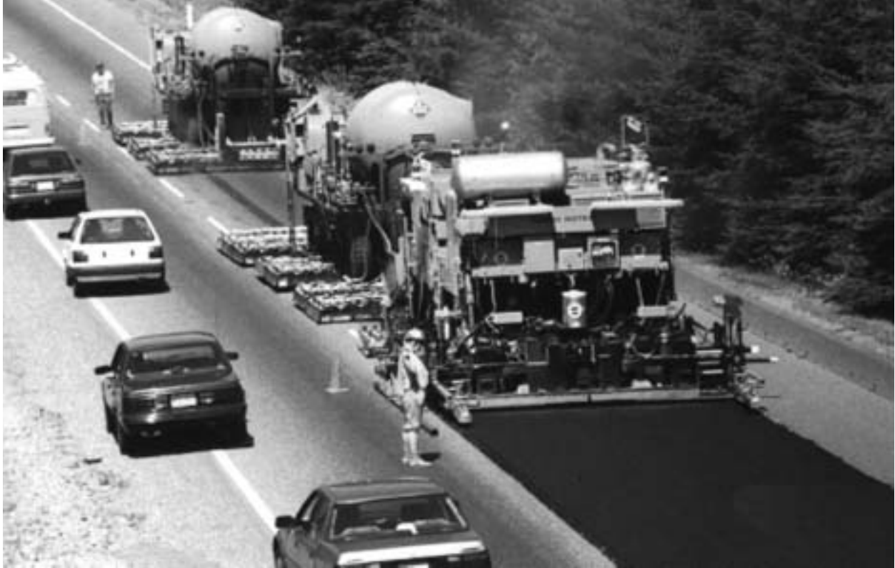
Figure 1-11: Single stage Remixing train
