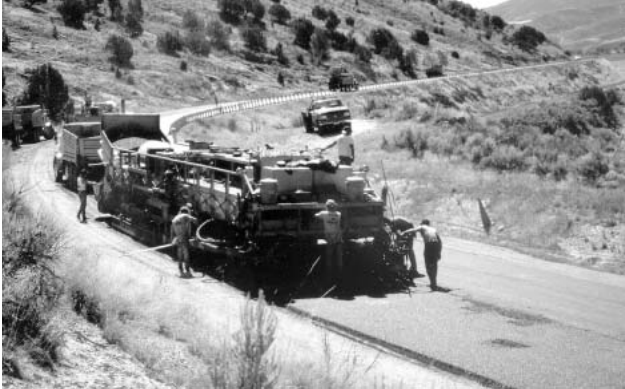
Figure 1-14: Single pass repaving
