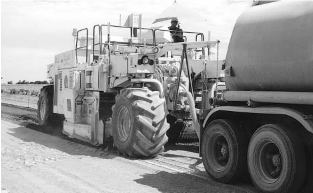
Figure 11-2: Chemical stabilization on rural roadway
