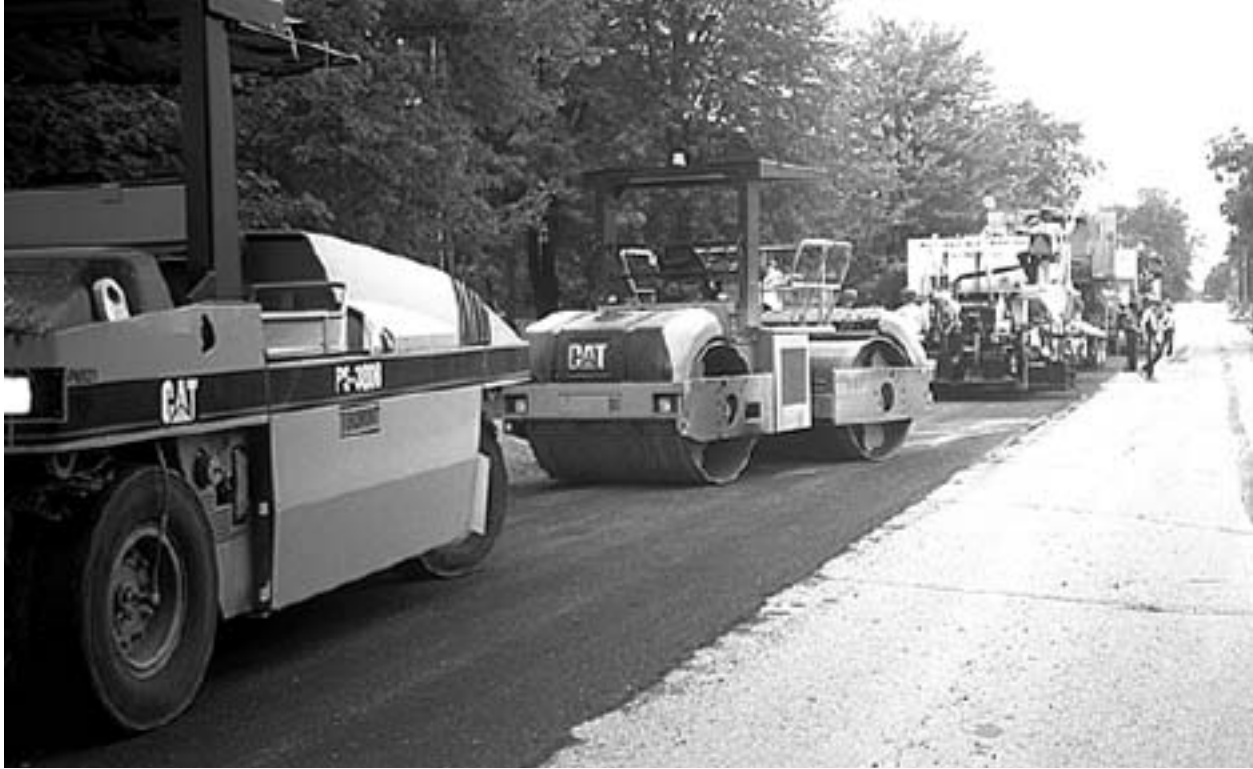
Figure 1-21: CIR compaction
