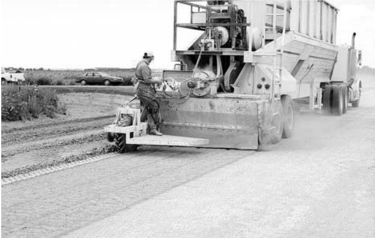
Figure 12-4: Dry stabilizing agent being spread prior to FDR
