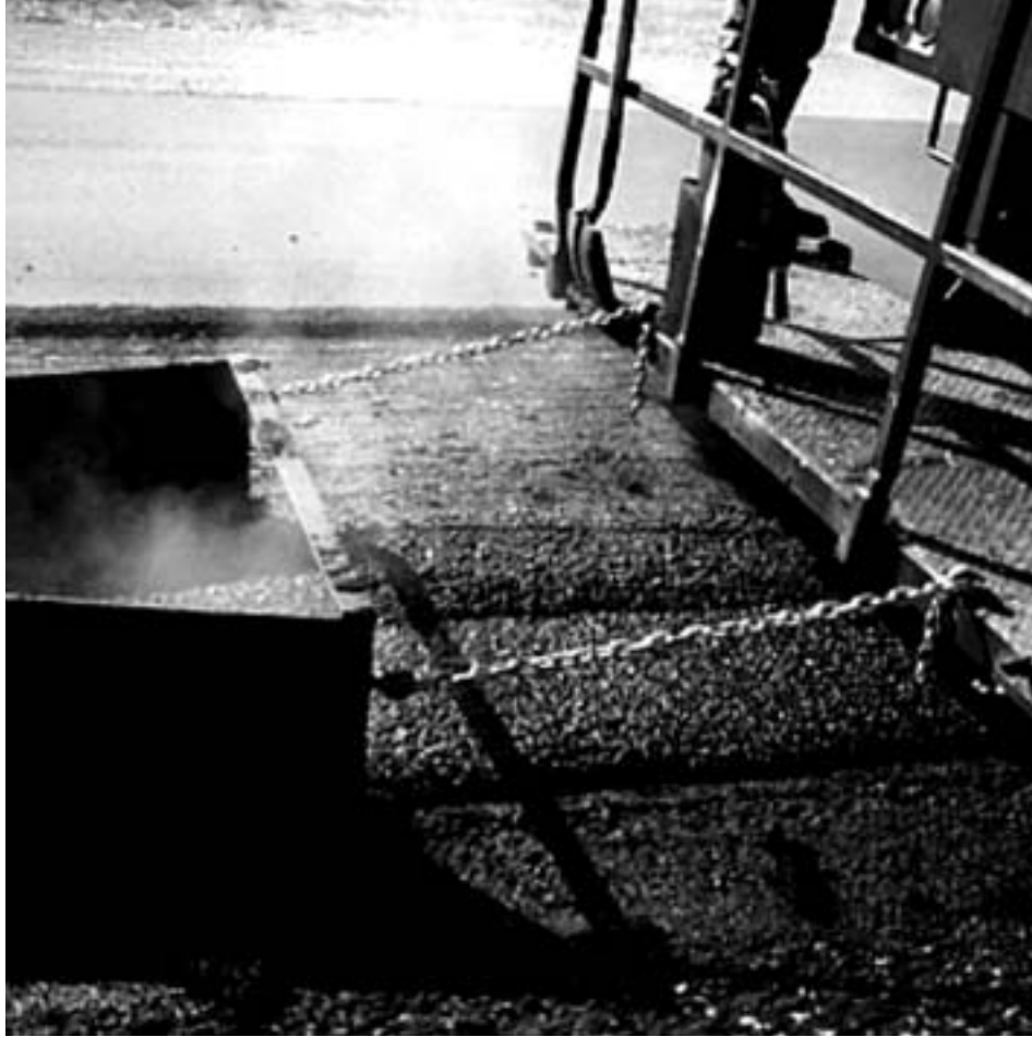
Figure 6-14: High fluids content in first layer of a multi stage project
