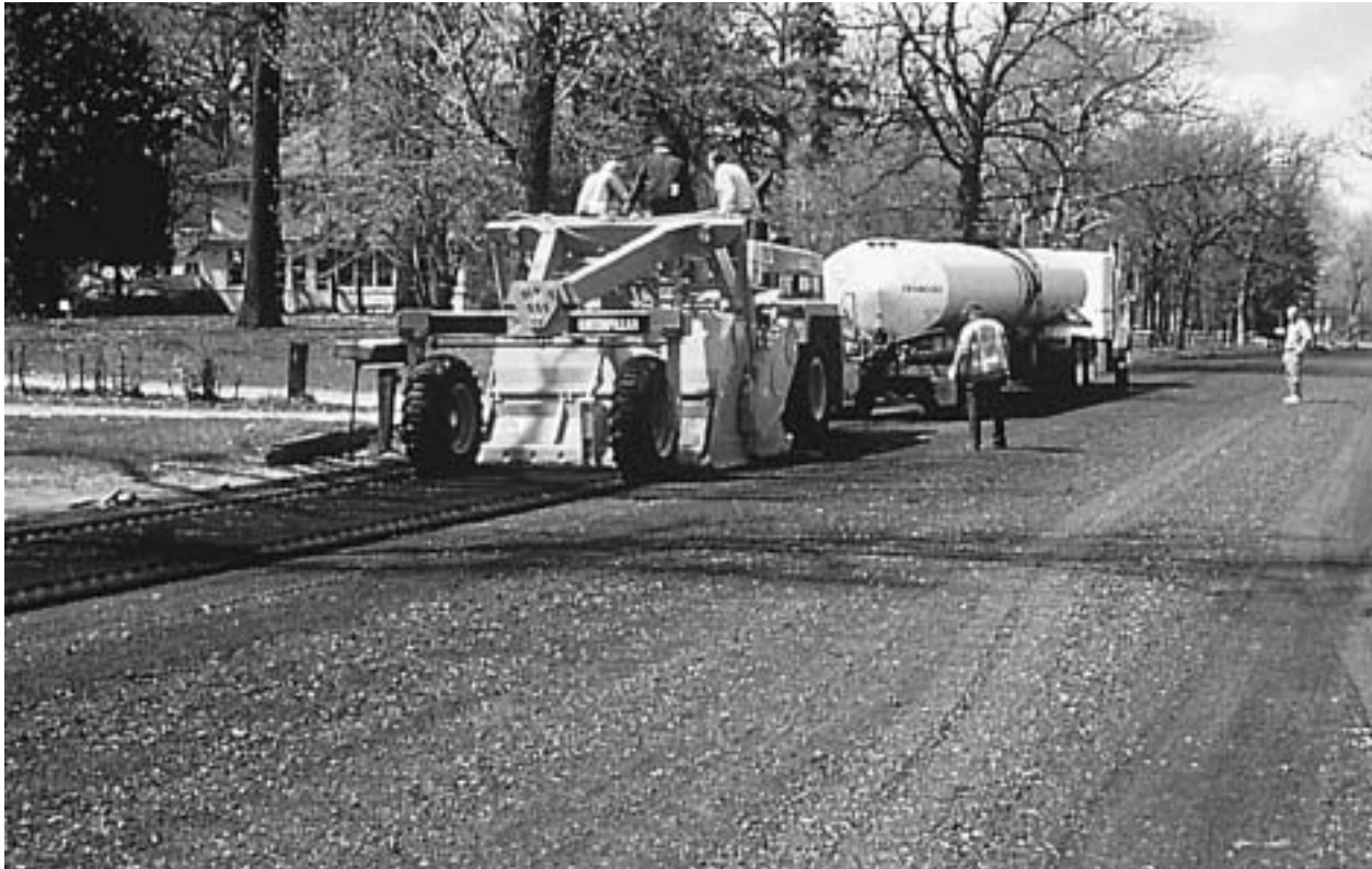
Figure 12-3: Reclaiming Operation
