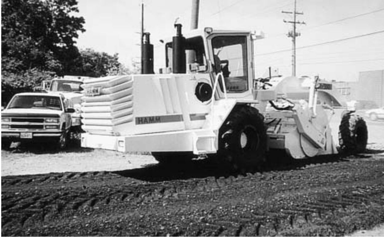
Figure 11-1: Mechanical stabilization with RAP as additive
