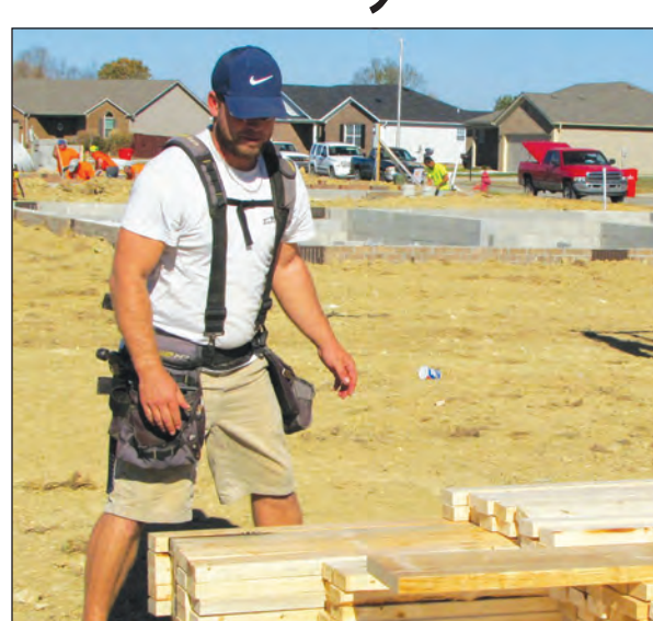
The City of Berea Planning and Codes Department is encouraging residents and contractors to be aware of deck safety during the month of May, Building Safety Month. Residents have several ways to check if their deck is safe.
