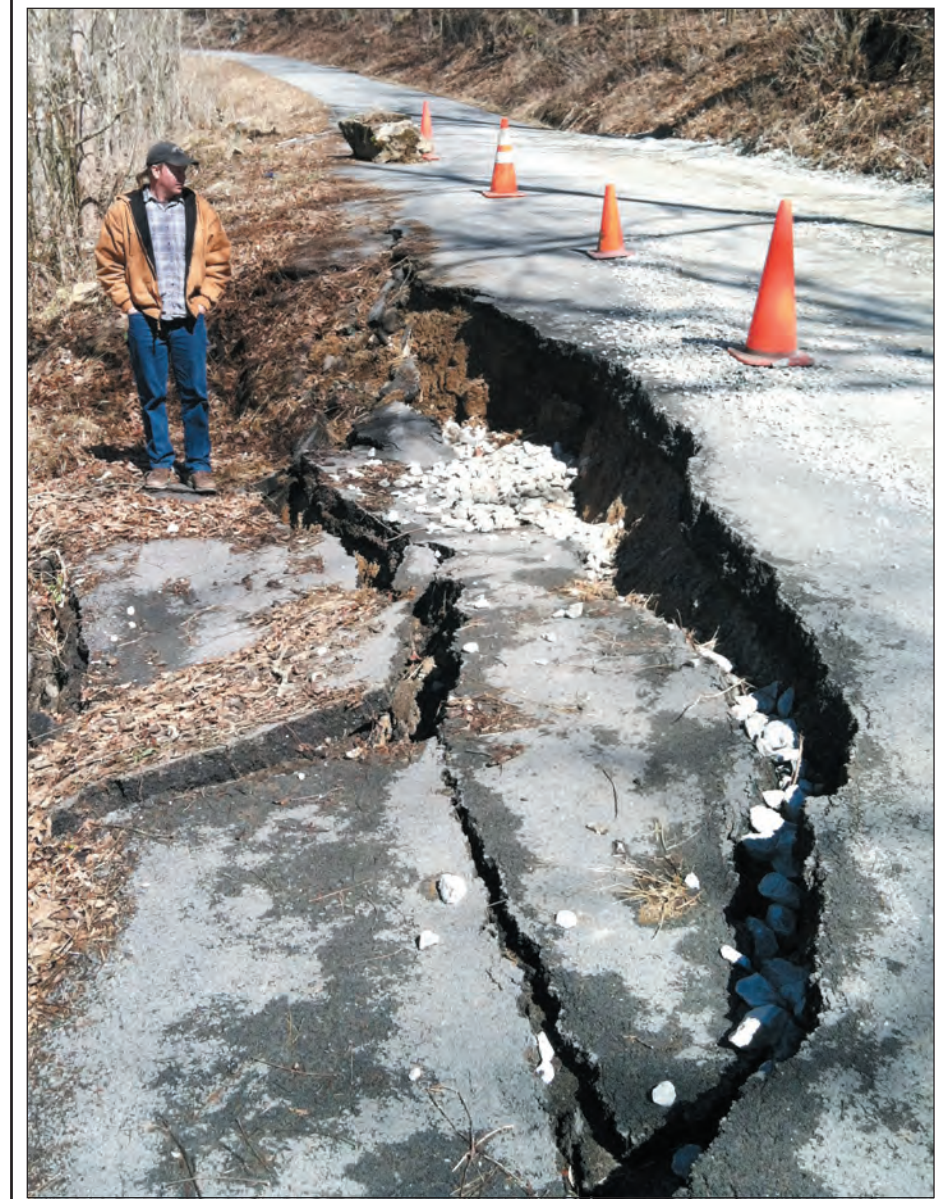
County Road Department workers finished repairing this slip on Lower River Road on Tuesday. The slip had closed the road for a week. Another slip, on Lambert Road, is awaiting an engineering design to be repaired but did not cause the road to have to be closed.
