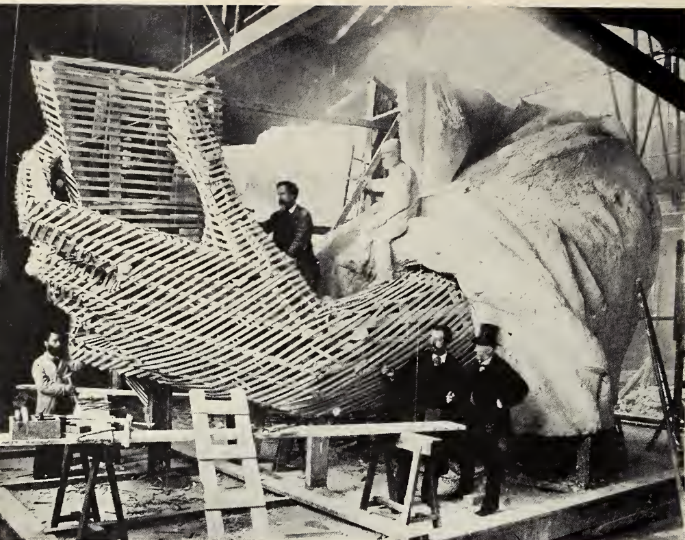
A French crew, under sculptor Bartholdi's orders, at work on a plaster cast of Liberty.
