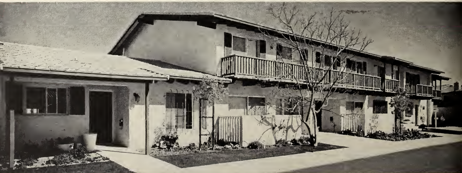
Loma Riviera Town Houses condominium in San Diego, Calif. To some, condominiums represent the ideal kind of housing.
