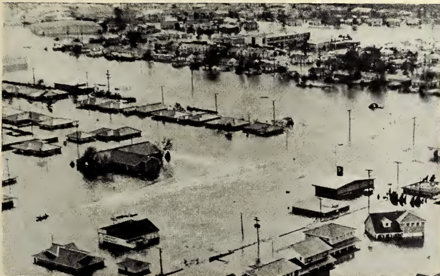
Hurricane Betsy's 150-mph winds felled trees and buildings and her accompanying floods left thousands homeless. One inundated area covered 300 square blocks. While wind damage is
