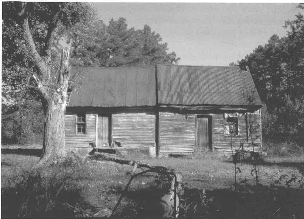
One-room-plan Houses — An example of two typical southern Delaware one-room-plan houses, joined together into a single structure at some point in their histories, survived into the early 1980s near the southwestern Sussex hamlet of Hearn's Crossroads, photo by Richard B. Carter, circa 1980.
