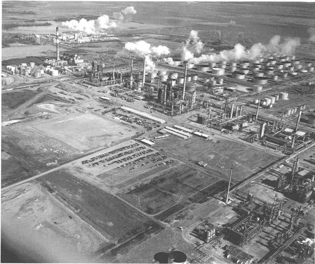
Oil Refinery — A 1981 aerial view of the Getty Oil Refinery complex near Delaware City, photo courtesy of the Delaware Economic Development Office.
