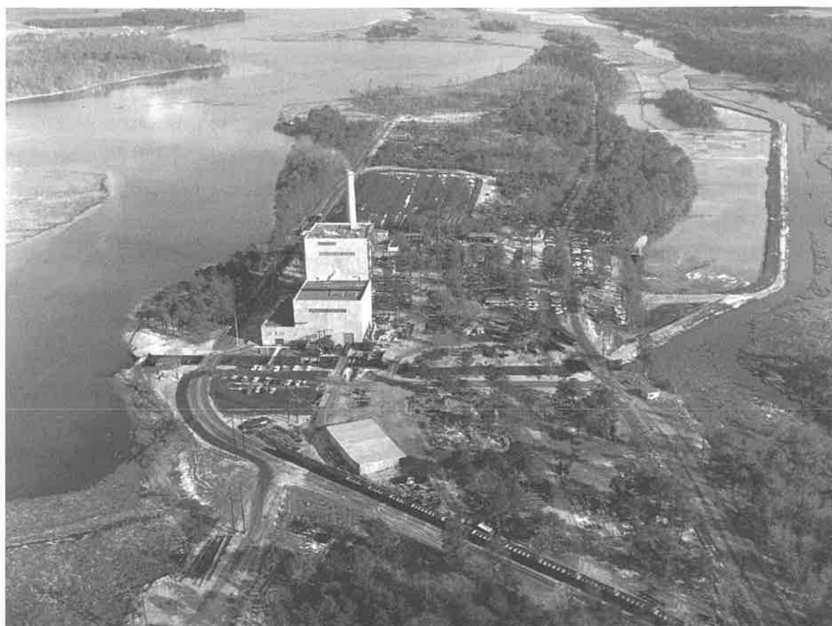
Power Plant — An aerial view of the first phase of the Indian River Power Plant as it appeared in 1957, soon after its construction. The plant has since been enlarged several times, courtesy of the Delaware Public Archives.
