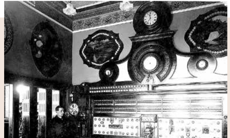
Watch room with telephone switch board. Photo DFES Collection.
