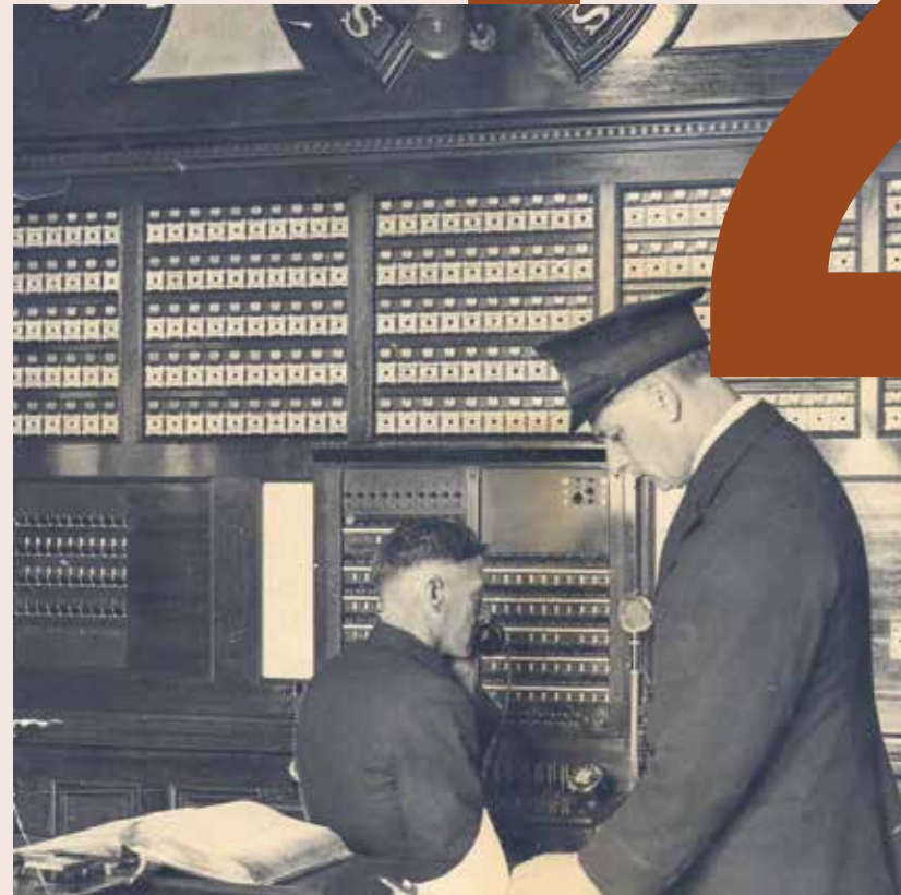
Watch room with telephone switch board behind duty watchman. Photo DFES Collection.
