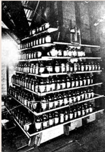
Batch of batteries that required regular servicing. Photo DFES Collection.
