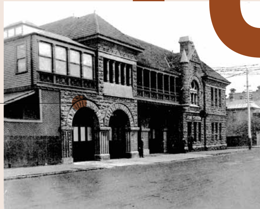
Fourth Engine Bay and Billiard Room Extension. Photo DFES Collection.
