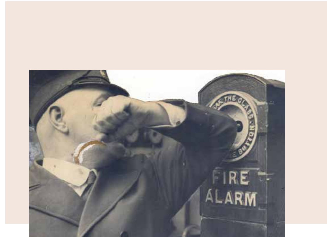
Fire alarm being activated above. Photo DFES Collection.
