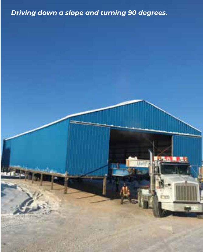
Pole shed is ready to go, loaded on their prime moving truck and scissor lifting dollies.
