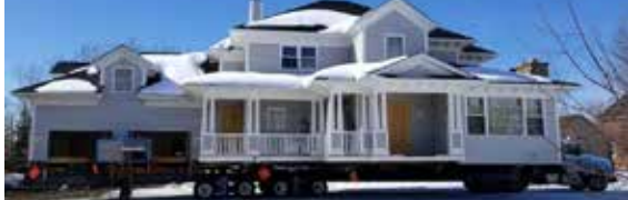
High River Flood House 2013. Was moved around 350 KM took 3 days to move as it was moved with 3 other houses.
