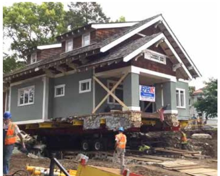
House being moved in South Minneapolis on power dollies.
