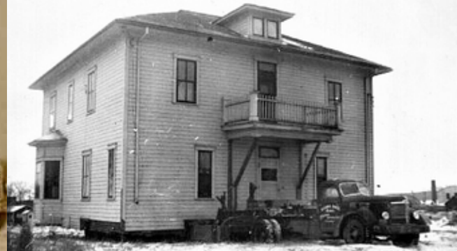
Wood timber beams used from 1953-1970, in the early years of Reimer Building Movers
