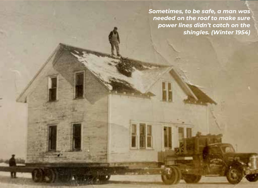
Large two story house pulled with the KB8. A double bunk was required to handle the weight of this house. The frame of the truck was sitting right down on the axle during this move due to the weight of the building. (Winter 1955)
