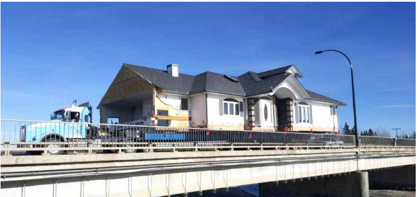
Ready to Move (RTM) home from Nelson's Homes. Building moved about 25km with just protective wrap and stuccoed on site.
