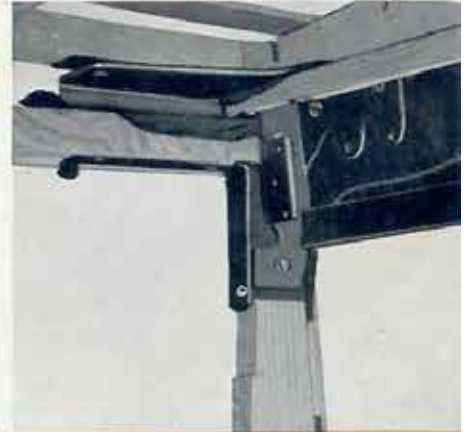
Front Corner Roof Brace
