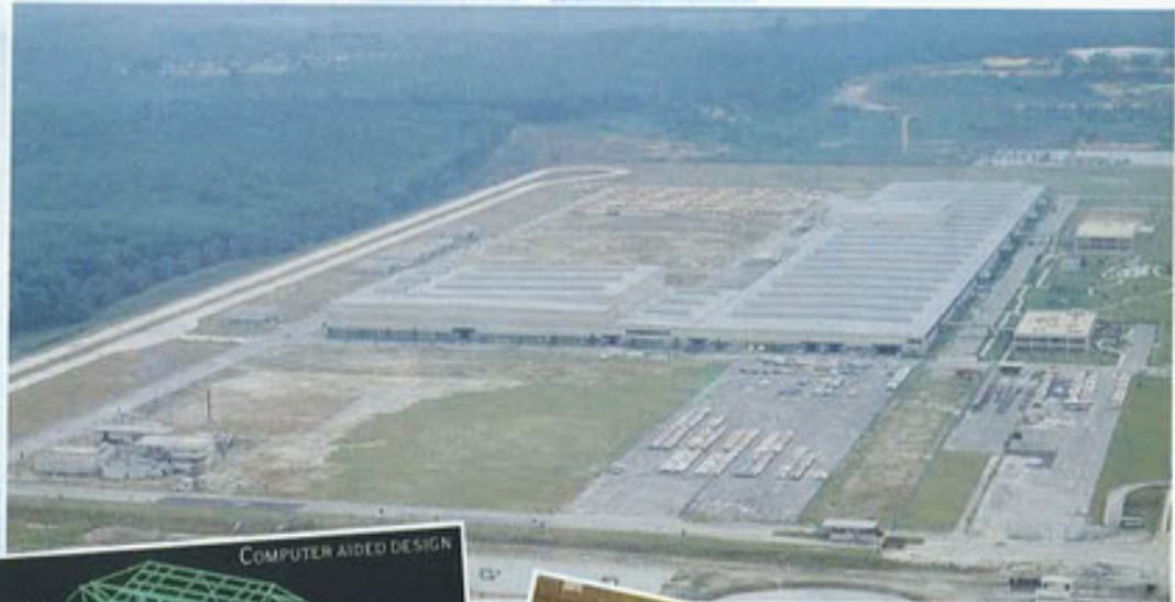
PROTON MANUFACTURING PLANT
