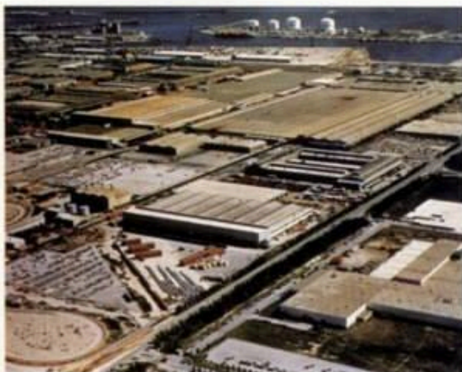
Zona Franca, Barcelona factory: Engines, coach-building, assembly.
