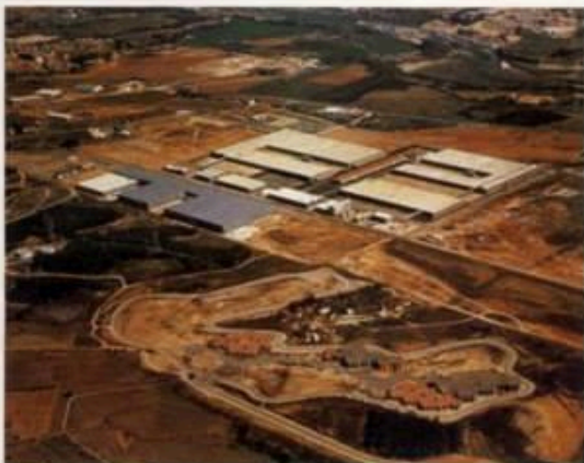
Martorell factory. Suspension, brakes and steering, spare parts warehouse, research and study center.
