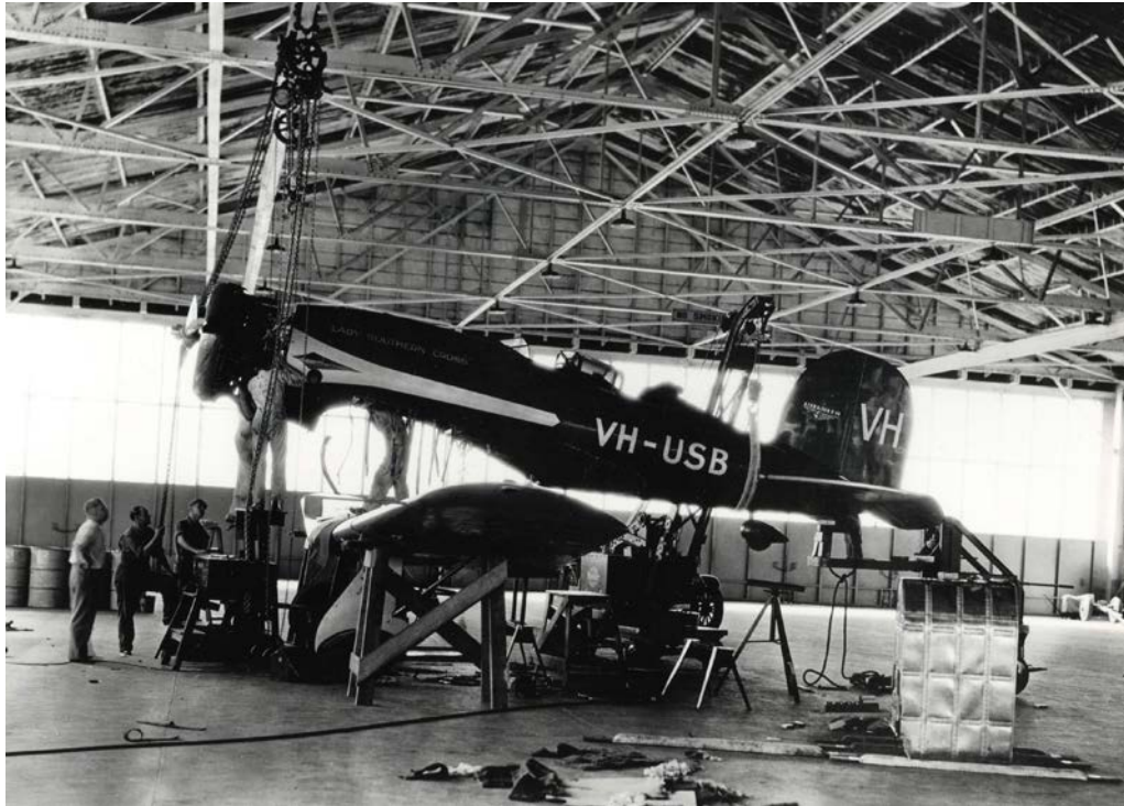
Fig. 72. Repairs to LADY SOUTHERN CROSS in Wheeler Field hangar November 2, 1934.
