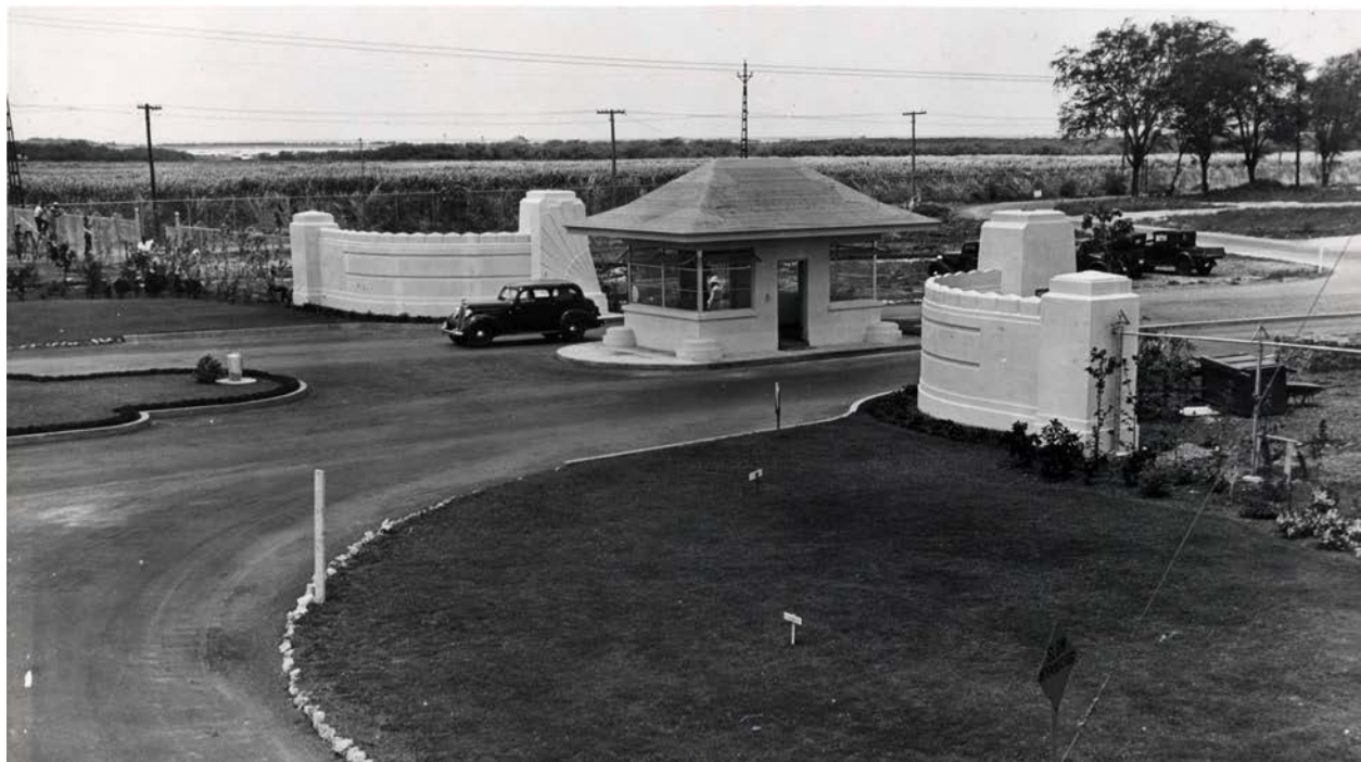
Fig. 99. Hickam's main entrance 1938.
