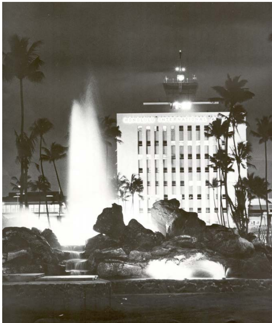
Fig. 135. John Rodgers Terminal, Honolulu International Airport, 1964.
