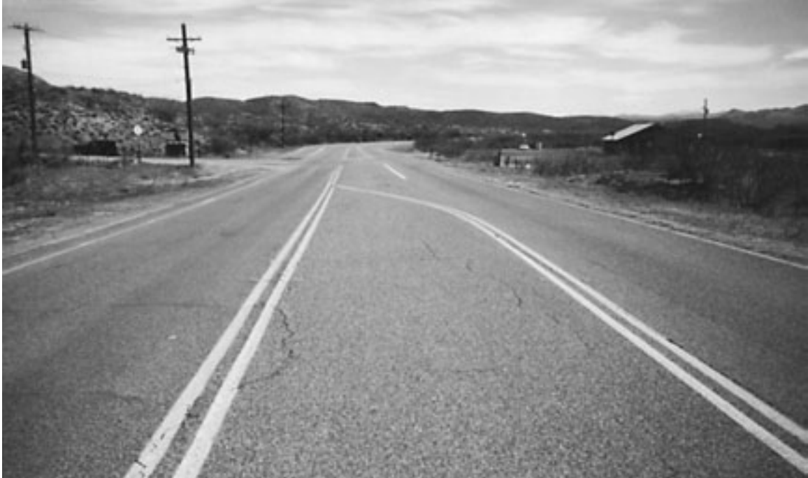
Figure 38. Segment of Old State Highway 73
