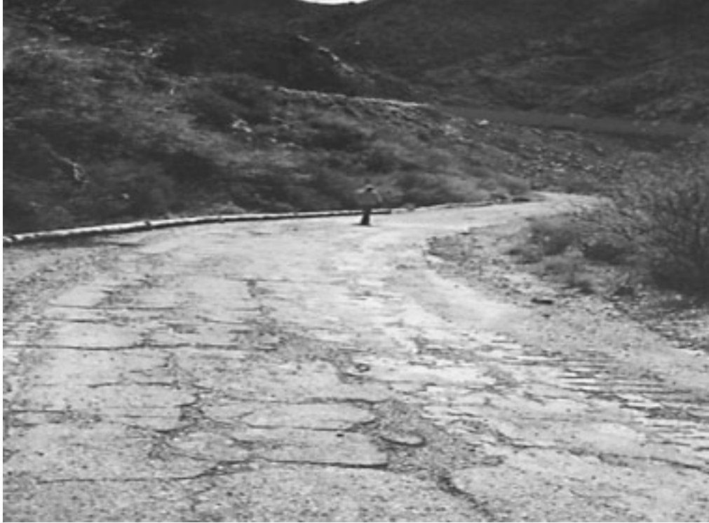
Figure 31. Abandoned Segment of U.S. Highway 60
