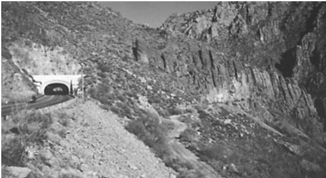
Figure 32. Abandoned Segment of U.S. Highway 60
