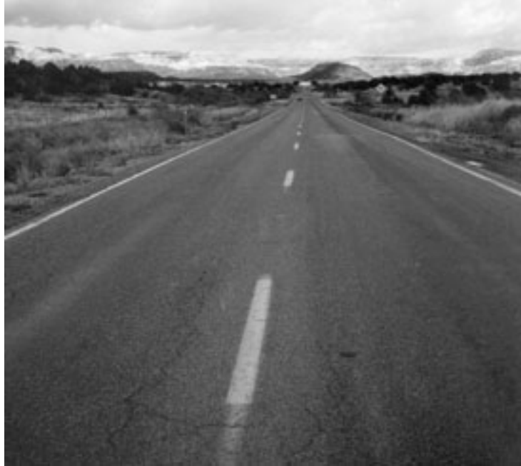
Figure 46. Segment of Old State Highway 79
