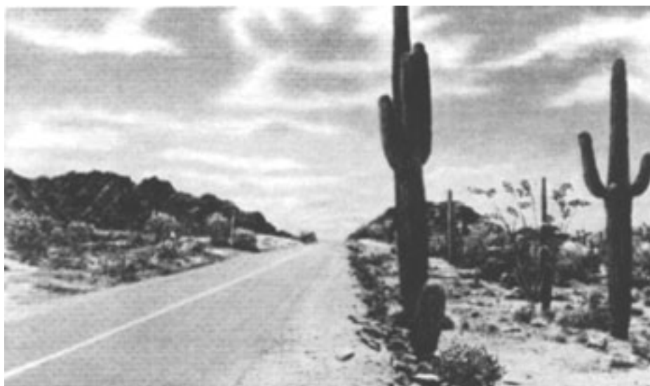
Figure 20. U.S. Highway 60 near Wickenburg, 1939
