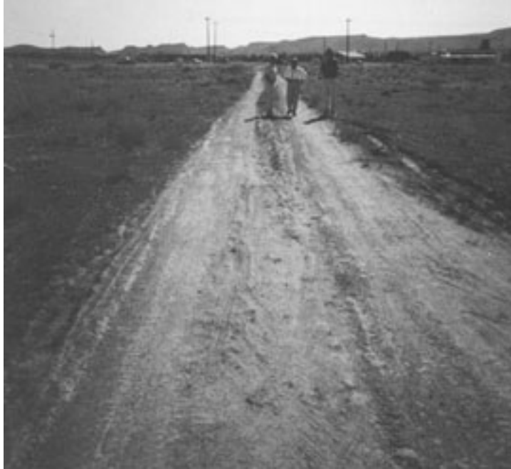
Figure 25. Segment of the Beale Wagon Road that Has Lost Integrity
