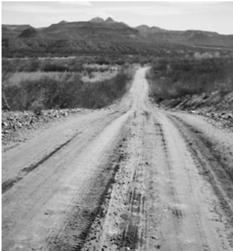
Figure 41. Segment of Old State Highway 73
