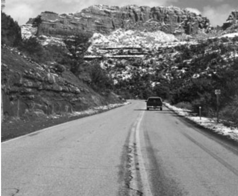
Figure 48. Old State Highway 79 at Lower End of Oak Creek Canyon
