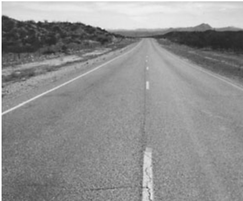
Figure 39. Segment of Old State Highway 73
