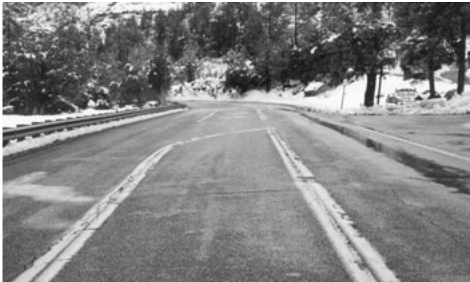
Figure 49. Segment of Old State Highway 79 in Middle Oak Creek Canyon
