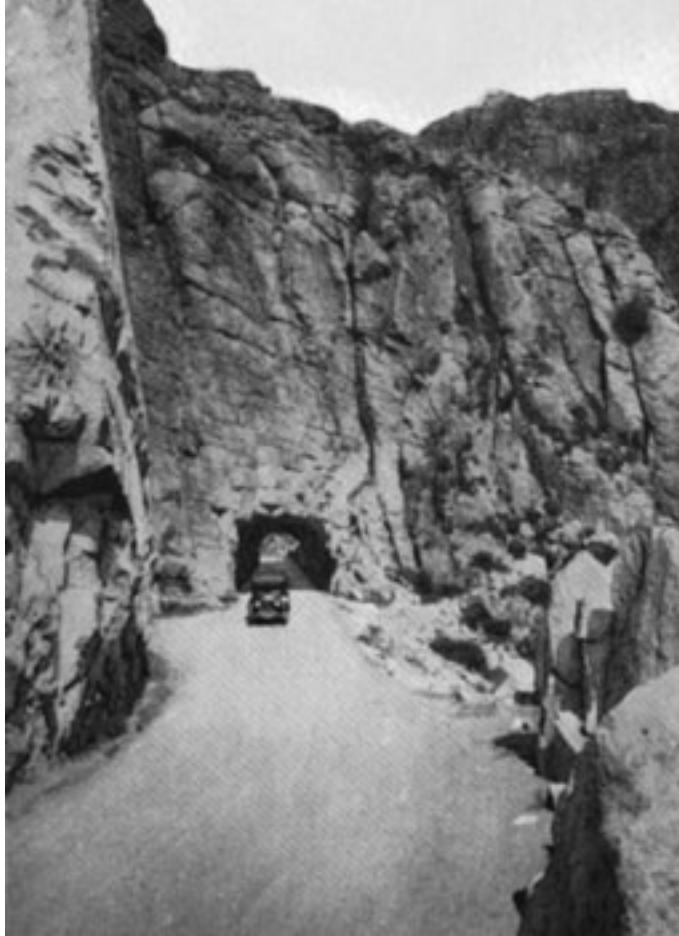
Figure 16. Claypool Tunnel on U.S. Highway 60, circa 1932
