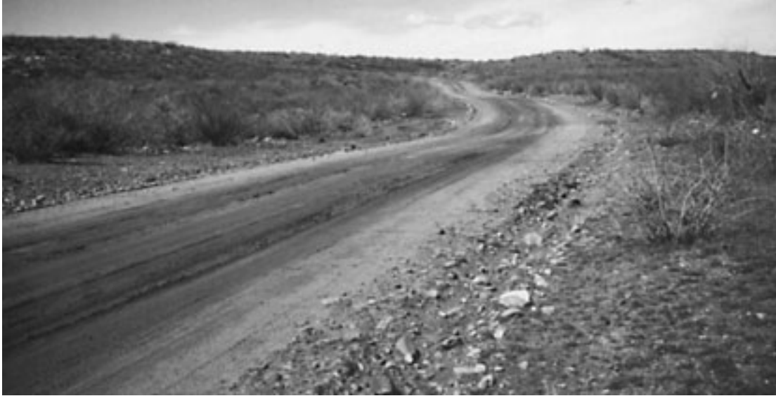
Figure 40. Segment of Old State Highway 73
