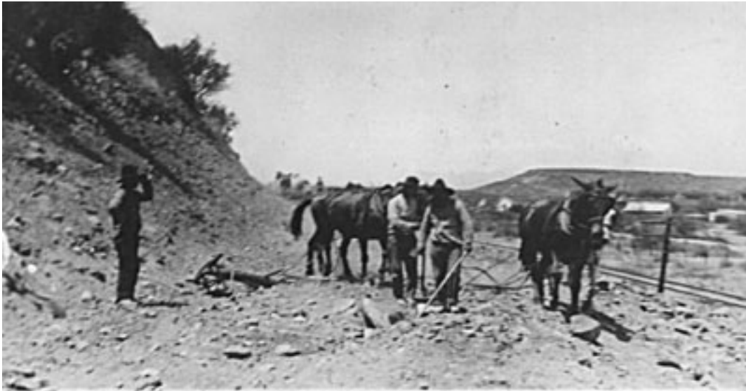
Figure 7. Mules in Arizona Road Construction, circa 1920
