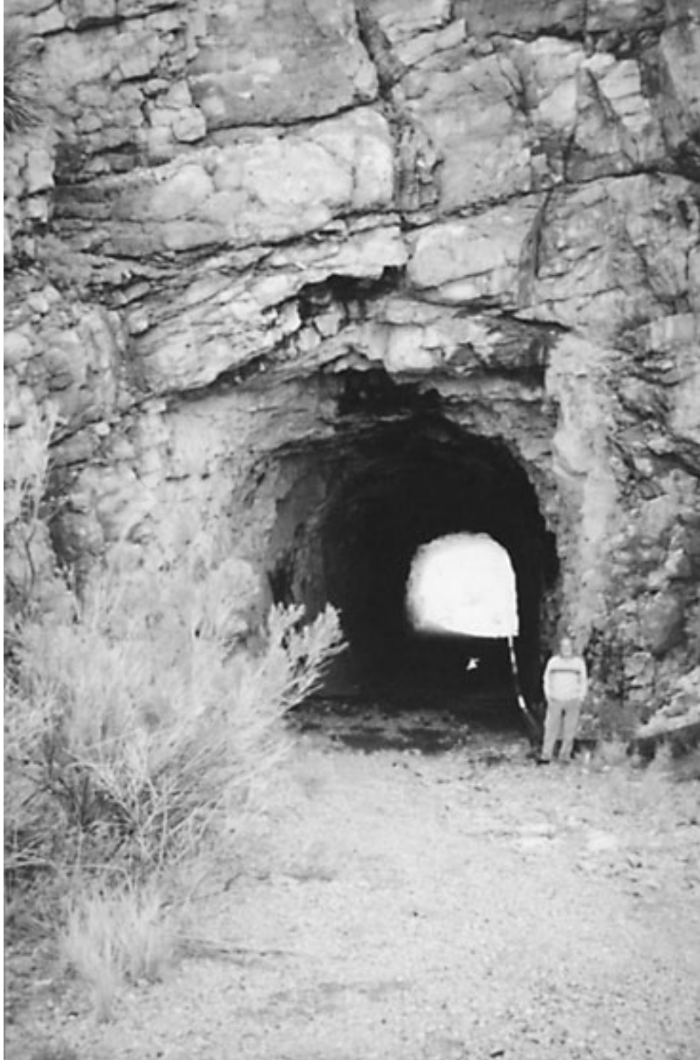
Figure 35. Claypool Tunnel along Abandoned Segment of U.S. Highway 60
