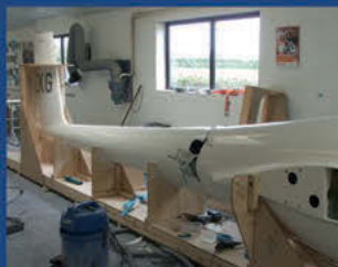
ASK21 in our Jig for fuselage repair
