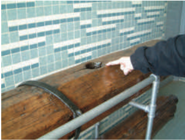
Figure 6 - Hole for fire plug.
