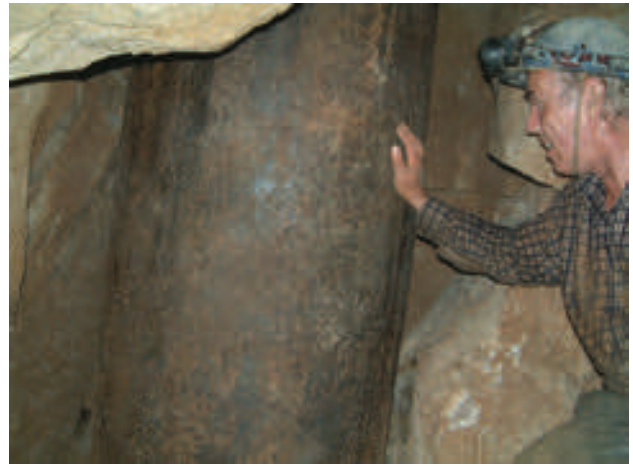
Figure 7 -Tony Waltham and caisson supporting low section of the Madison County Courthouse.
