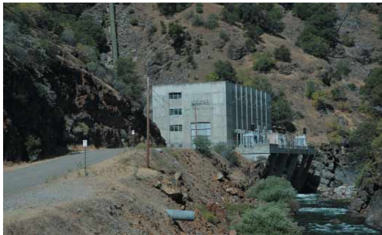
Top: The SFPUC’s Kirkwood Powerhouse generates electricity using water that flows from Hetch Hetchy Reservoir via the Canyon Tunnel. With modifications to the tunnel, Kirkwood could continue to produce nearly two thirds of its current output under a restoration scenario. Otherwise Kirkwood would become inoperable and have to be retired. Bottom: The Dion R. Holm Powerhouse, which produces about 40 percent of the SFPUC system’s annual hydropower output, would be unaffected by restoration of Hetch Hetchy Valley. It generates energy using water from two of the Tuolumne’s tributaries, Cherry and Eleanor Creeks.
