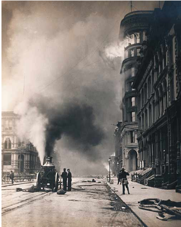
The 1906 earthquake's damage to San Francisco's pipes—not any inadequacies in its reservoirs—resulted in a lack of water to fight the devastating fire.
