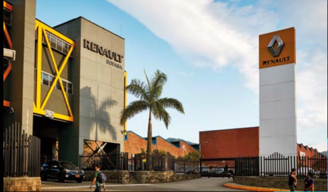
ENVIGADO SOFASA PLANT IN MEDELLIN, COLOMBIA
