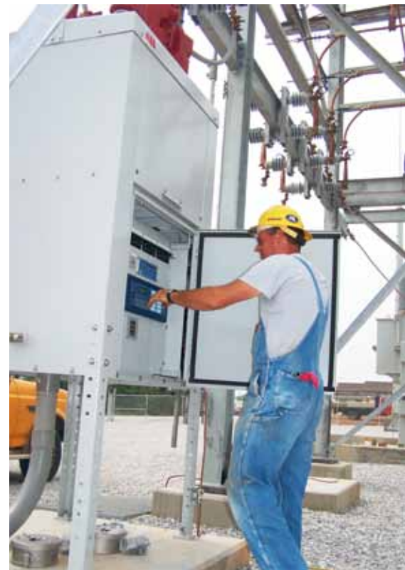
BELOW: Vince Weatherly at work on the new Republic Substation.
