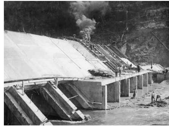
ABOVE & BELOW: Powersite Dam under construction.
