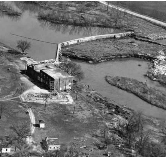
ABOVE: Grand Falls Power Plant, 1939.
