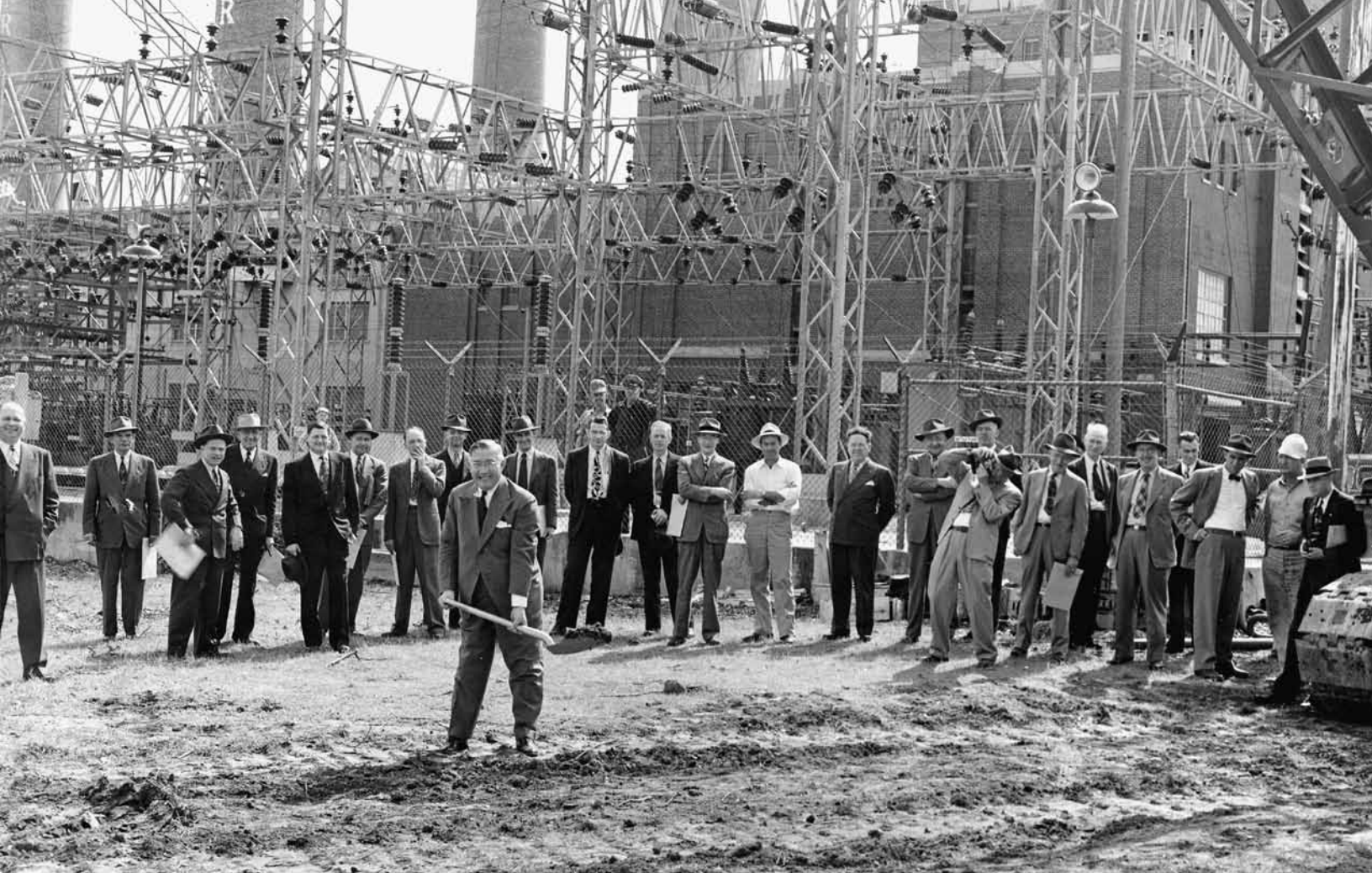
ABOVE: At 2:30 p.m., April 22, 1948, James E. Harsh, Chairman of the Board, pushed the cutting edge of a gold-plated shovel into the earth at Riverton symbolizing the start of construction of the $4,600,000 Riverton power plant. Riverton ground-breaking photo taken in 1948 includes three Empire presidents: Harsh with the shovel, McKee at far left and Drewelow fifth from the left.
