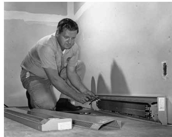
BELOW RIGHT: Gary Hilton installs baseboard heating unit in the 1960s.
